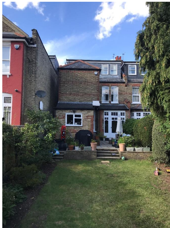
Rear of application site
