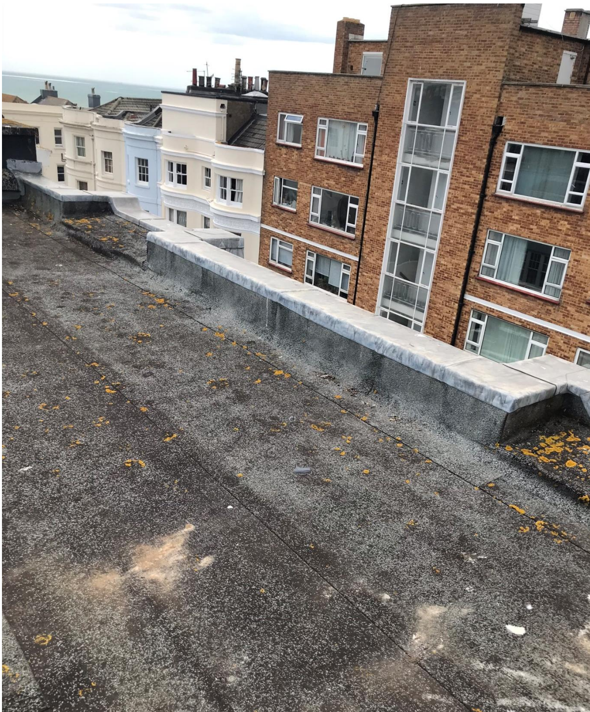
PHOTO 05 Existing flat roof view twds front (street)
