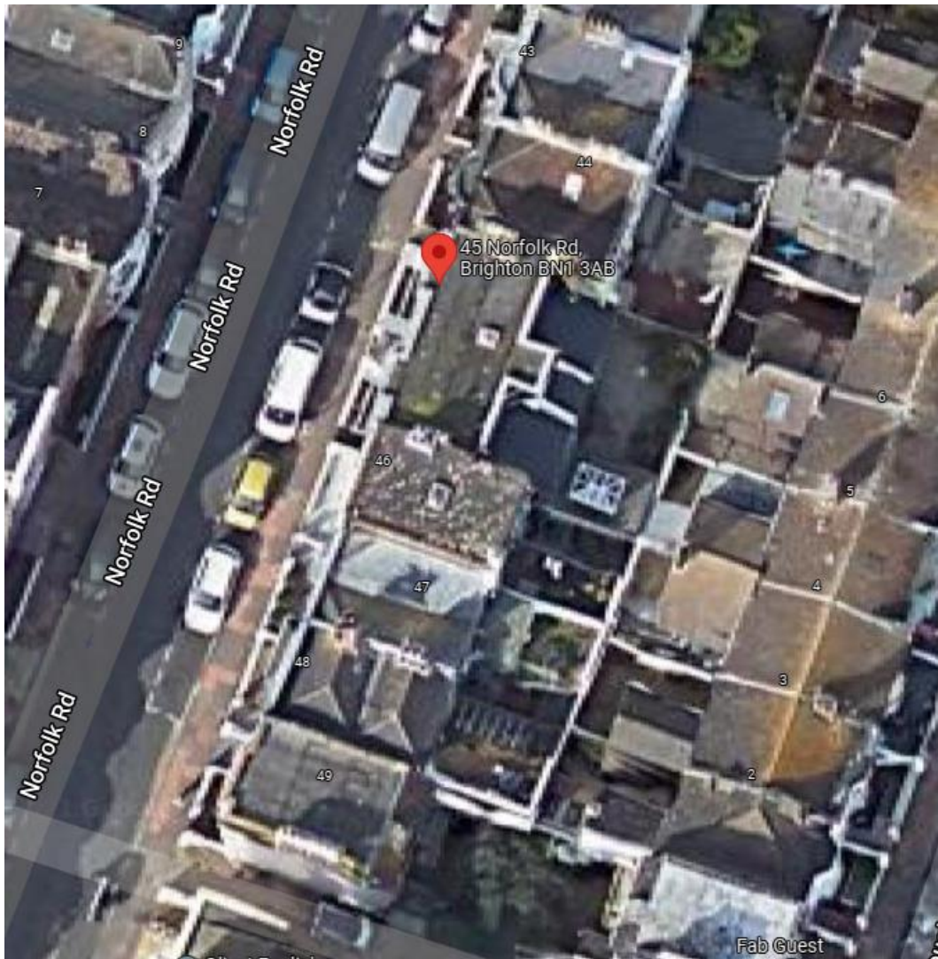
Aerial View Illustrating number 45 stair outcrop and alignment of adjacent facades
