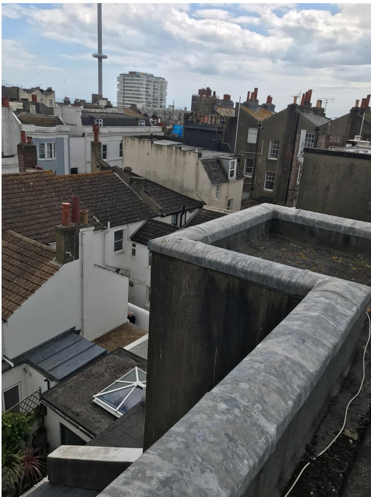
PHOTO 06 View from roof illustrating limited overlooking Heritage Statement – 45 Norfolk Road, Brighton BN1 3AB Installation of AC Unit to Planning Approved Roof Terrace
