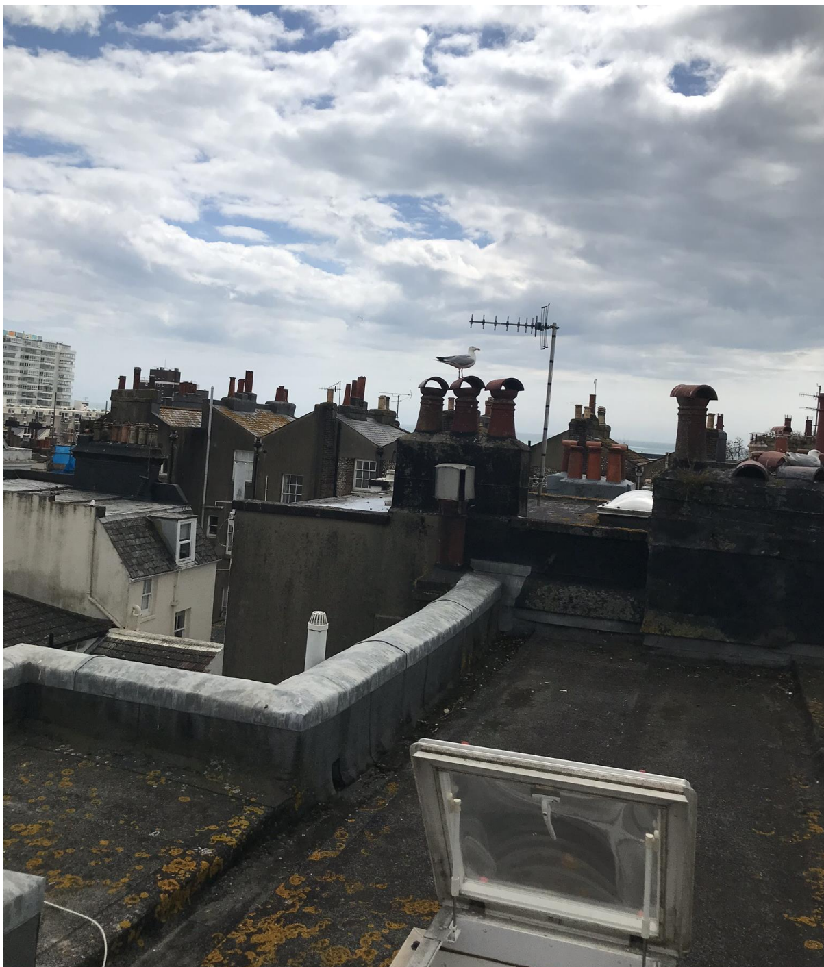
PHOTO 04 Existing flat roof view twds rear showing existing access hatch
