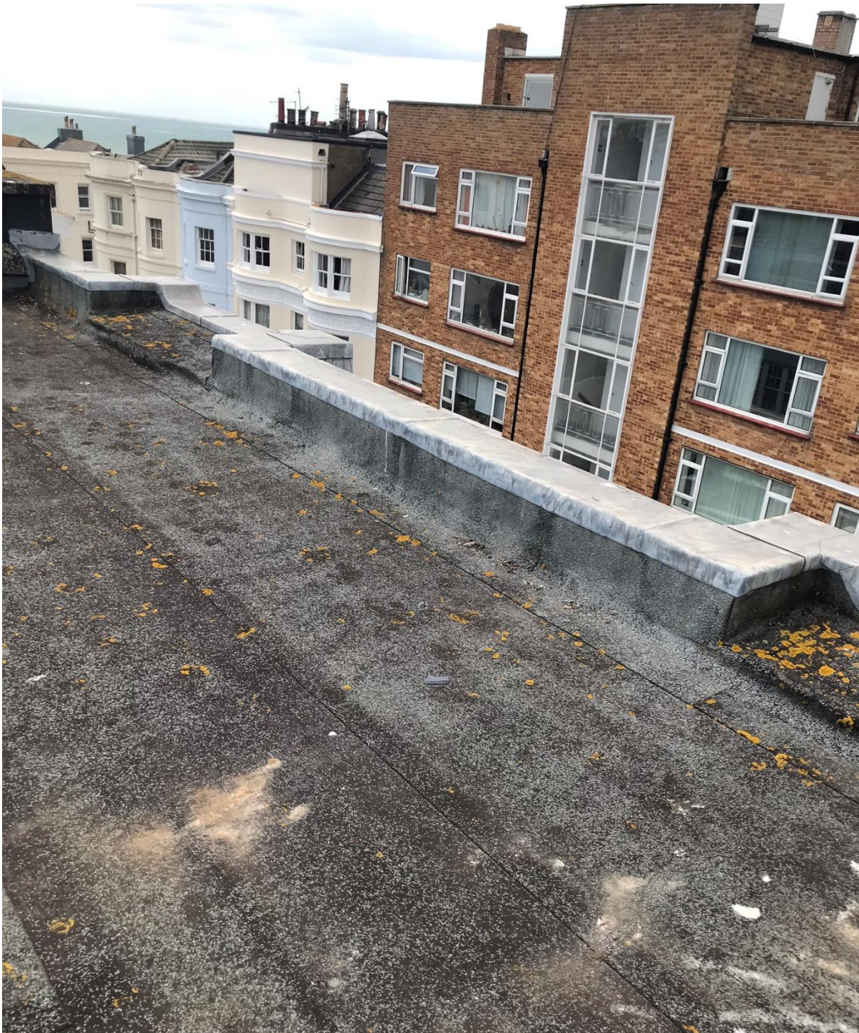
PHOTO 05 Existing flat roof view twds front (street)
