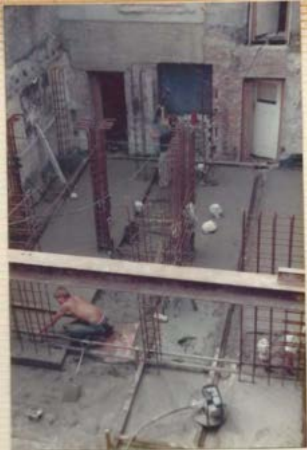
Basement: Raft, & Column & Wall Reinforcement in position, July 1978 (viewed from north)
