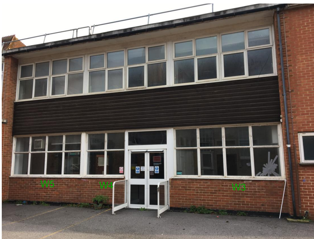
West Elevation Windows W3-W5 inclusive
