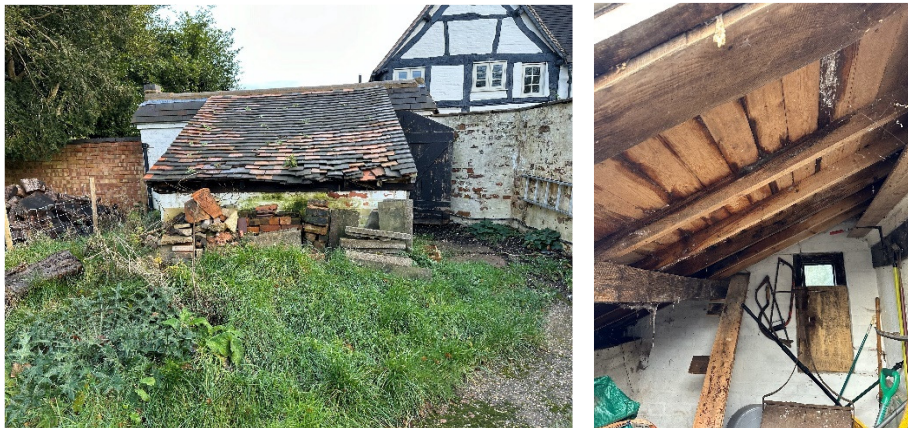
Photo of shed internally and externally – showing modern roof construction
