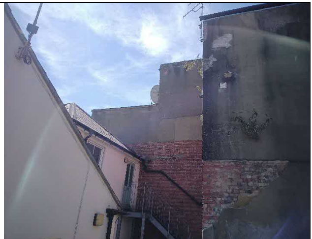
Photograph 2: Flat roof section of building
