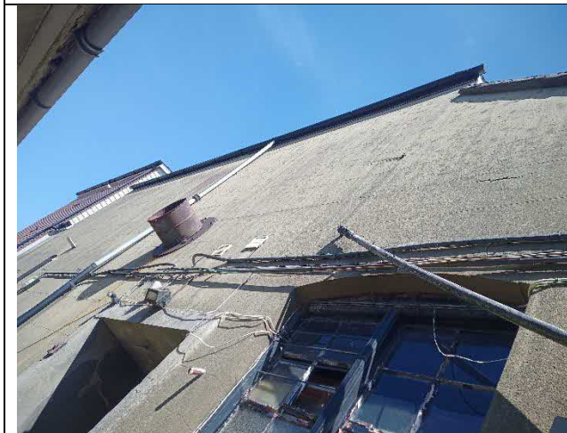
Photograph 3: West-facing rendered wall in which windows are proposed for installation
