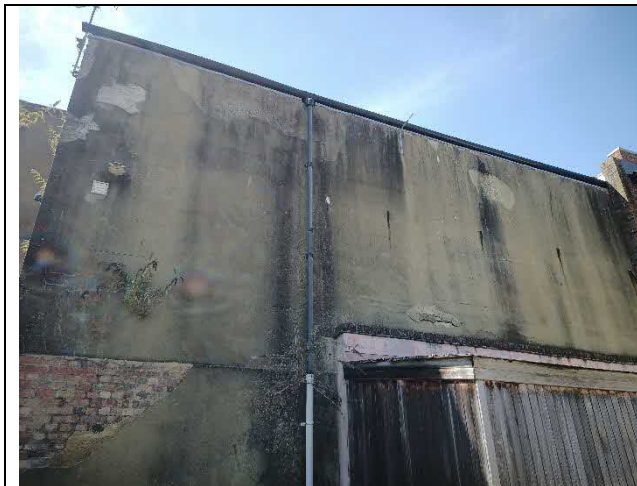
Photograph 1: East-facing rendered wall in which windows are proposed for installation
