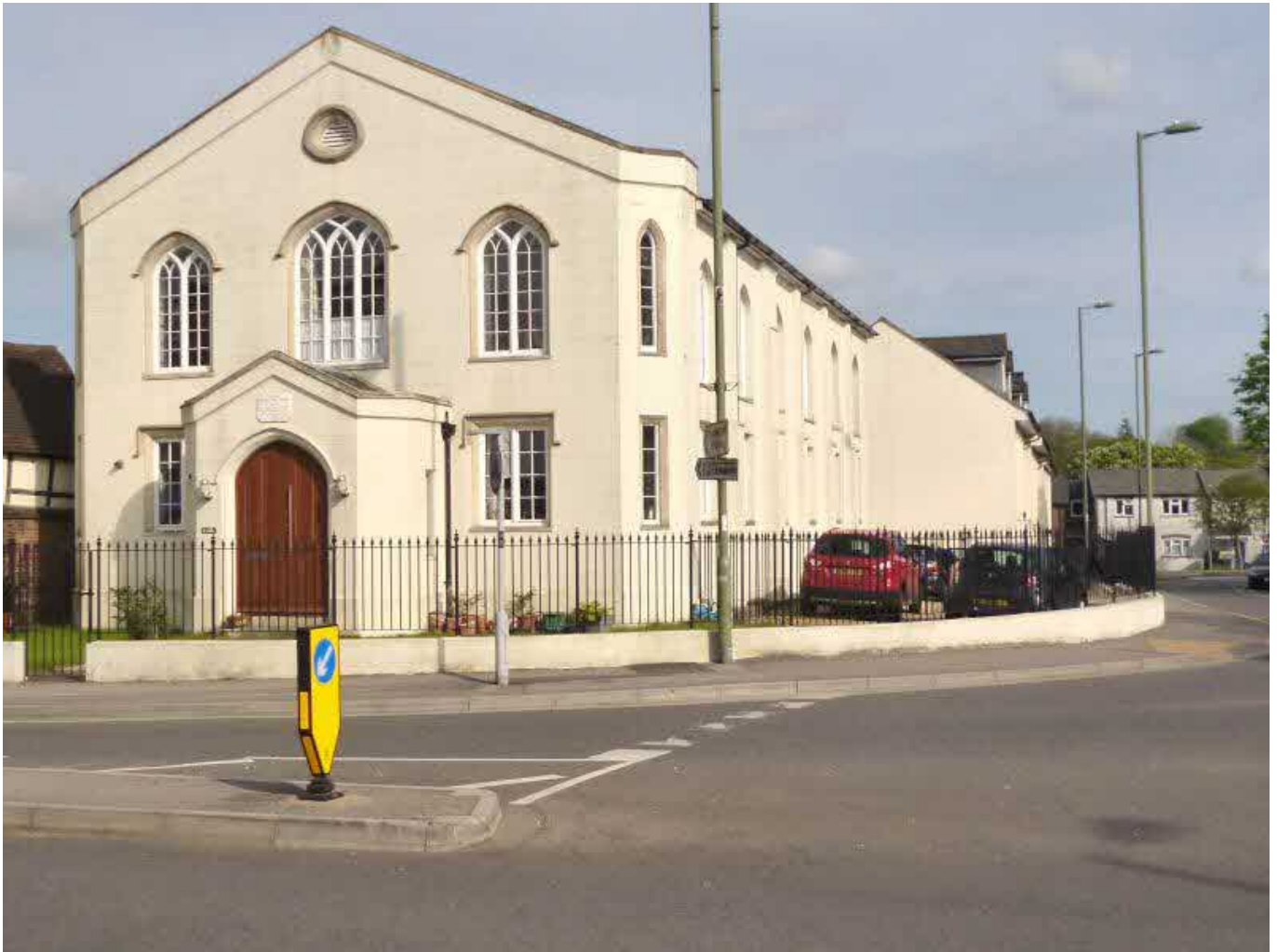
3. View of The Chapel
