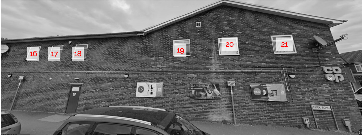
14 Station Road (Side Elevation)
