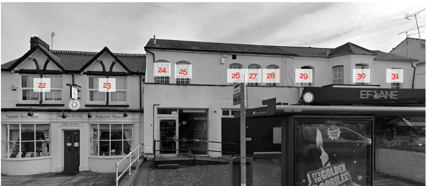
25 – 29 Station Road (Front Elevation)
