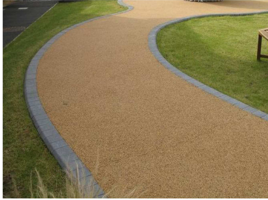
RESIN BOUNDED GRAVEL PAVEMENT
