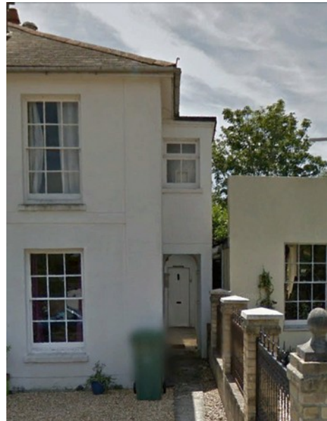
Image 4: Photo taken from Google Earth showing the property before the works were undertaken on the porch and the front door
