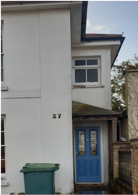
Image 3: Showing the porch and the front door currently
