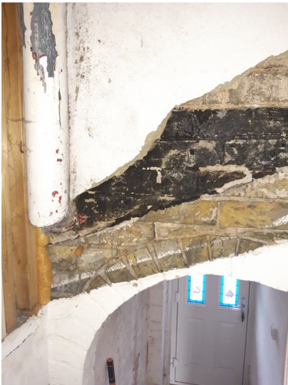
Image 7: Showing evidence of the former lean-to roof marked on the wall.
