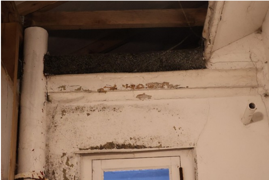
Image 8: Showing the engineered roof and the flat roof still in situ
