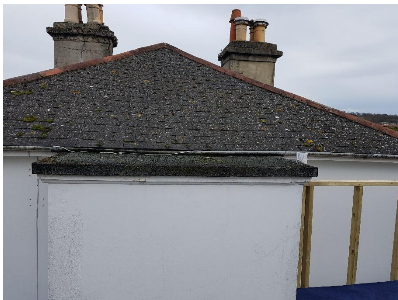
Photograph 7: Studwork for the new infill extension being constructed.
