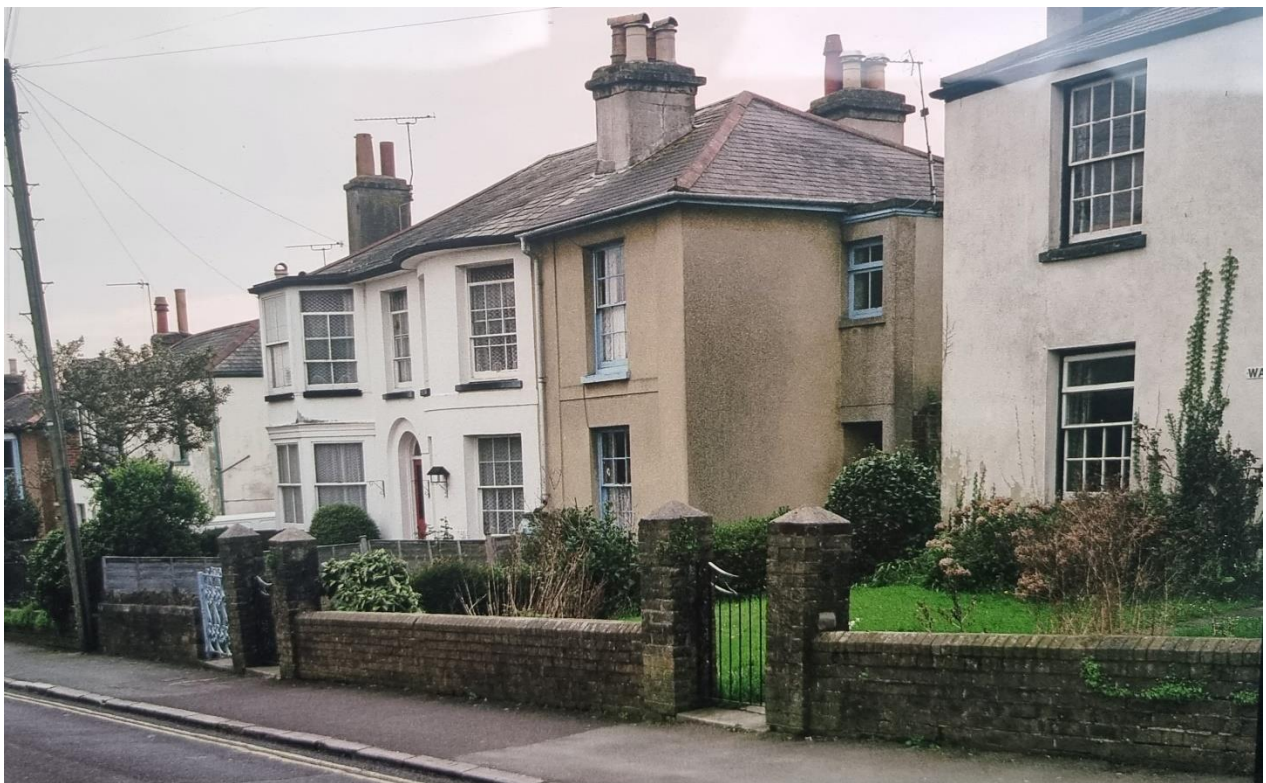
Photograph 1: 37 Melville Road in the 1960's-70's. The exterior finish is relatively new although has signs of weathering. Note the different roof tiles and the consistent render finish of the stacks. At this time the boundary between 37 and the house to the right was low and green.
