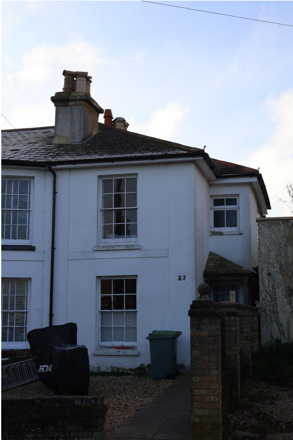
Photograph 2: The front elevation with the small pyramidal hipped porch roof on a simple timber support in the re-entrant angle between the earlier part of the house and the later added entrance extension. Photograph by the author 2023
