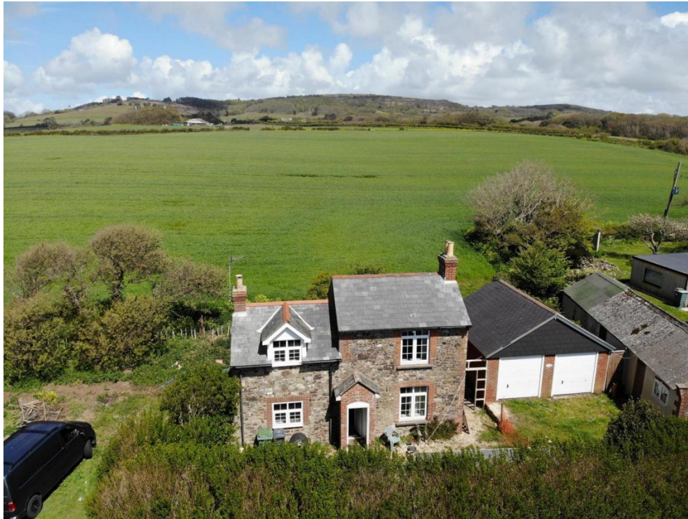
Aerial shot of the South side of the property.
