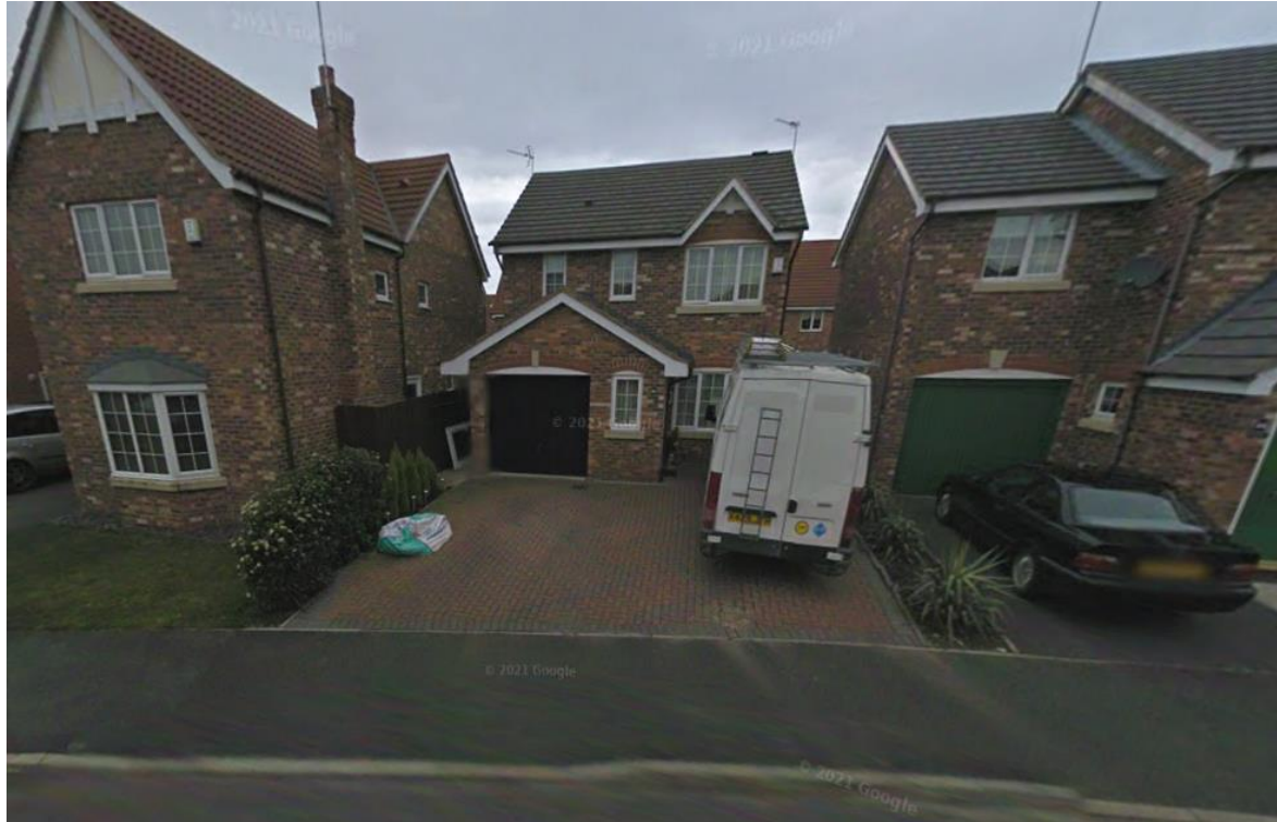
Photo 1: March 2009 (Google Street View)
