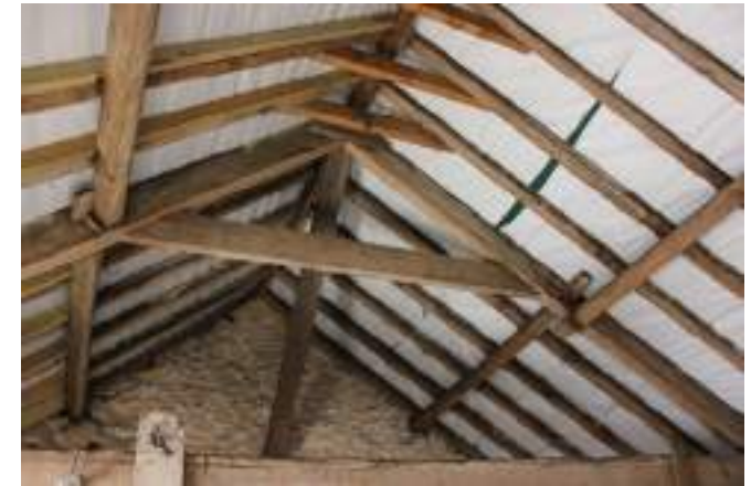
Collared truss with pegged purlins
