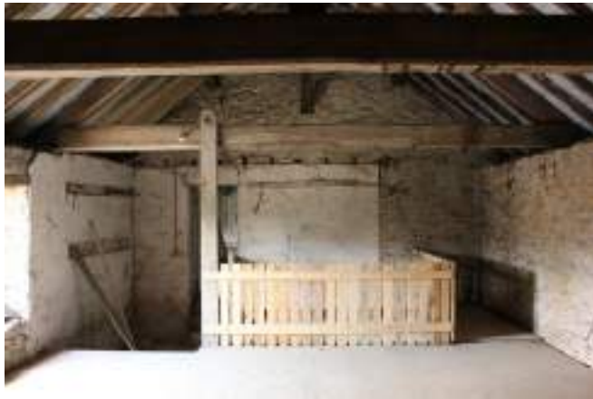
Stair with plastered walls to former enclosure
