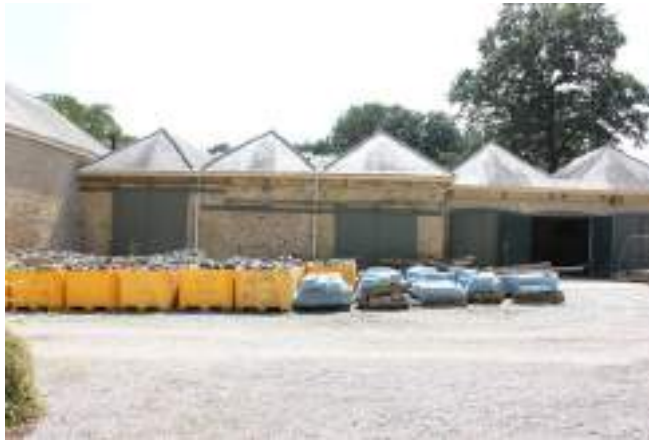
South courtyard range
