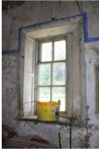
Stable window with bolection moulded architrave
