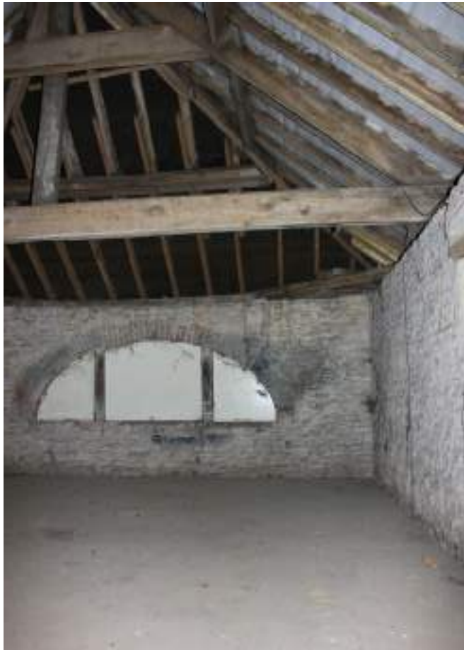
Hay loft or feed store with blocked Diocletian window with brick arch and stone mullions
