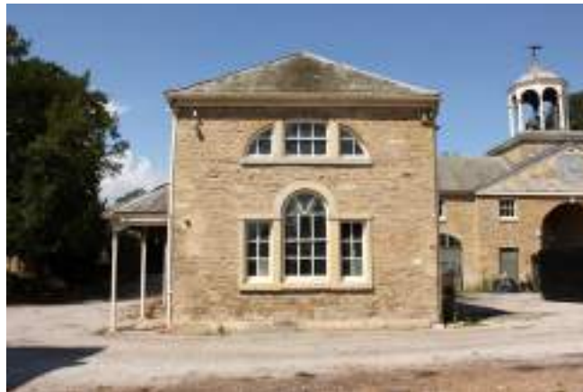
South wing gable end
