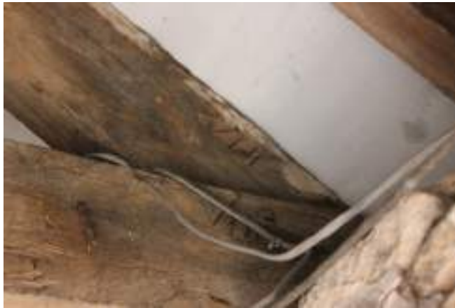
Carpenters marks to aid assembly
