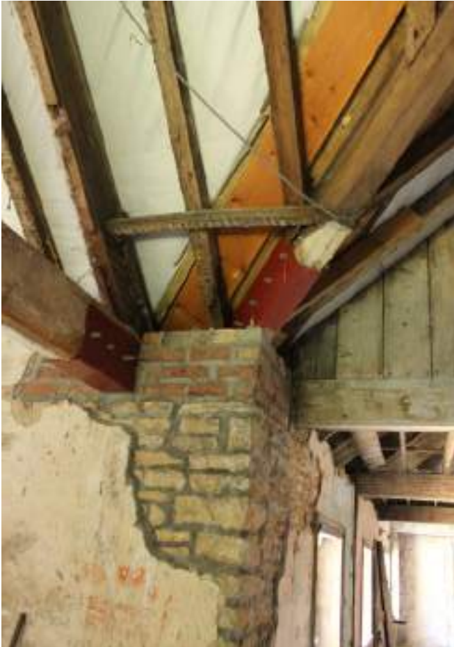
Modern roof repairs
