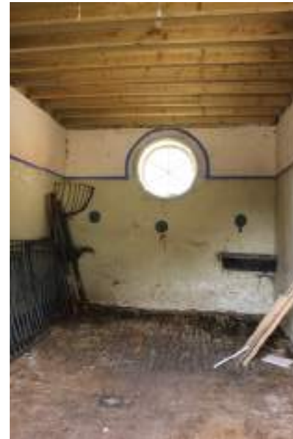
Loose box, south wing
