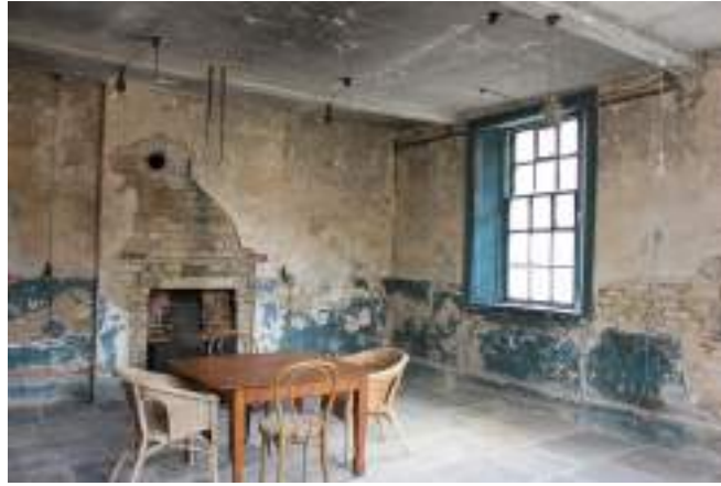
Possible former servants hall or laundry
