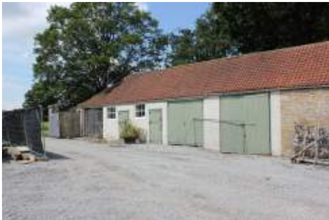
Single storey north range
