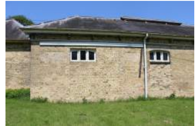
South elevation evidencing a series of historical modifications to earlier openings
