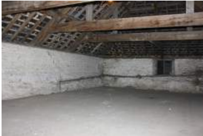
Loft above western extension, looking north
