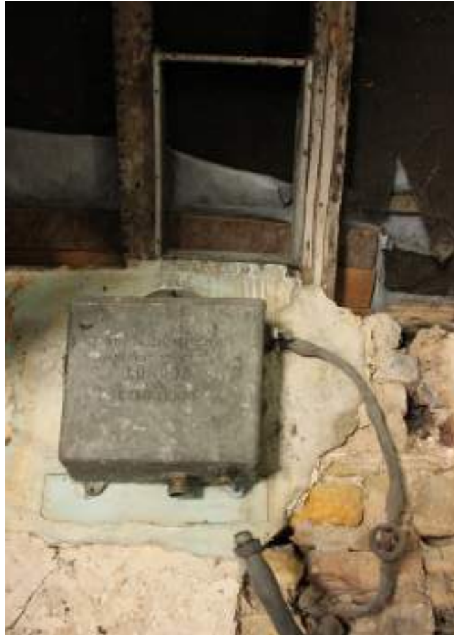
Early 20th century toilet cistern and roof light
