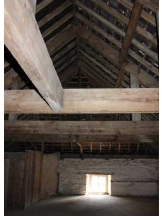
Loft above western extension, looking south
