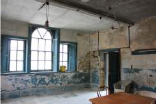
Venetian windows to possible former servants room or laundry
