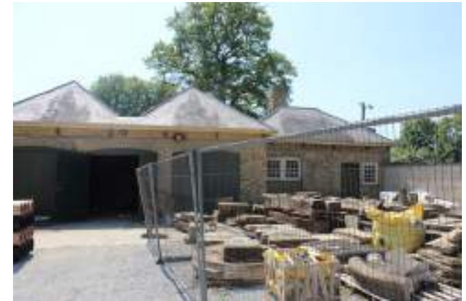
Westernmost building to courtyard
