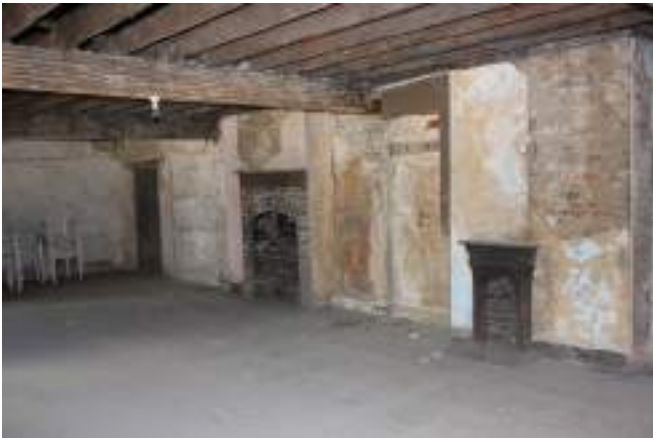
North wall with fireplace and range
