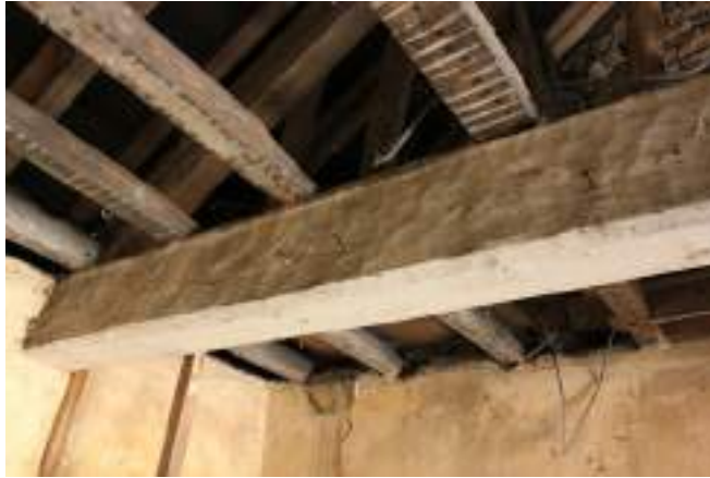
Ceiling beam with chamfer and hand tooled finish
