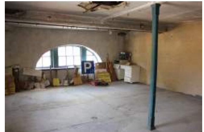
Room above former laundry
