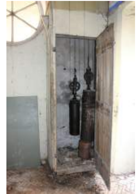
Clock weights in loose box
