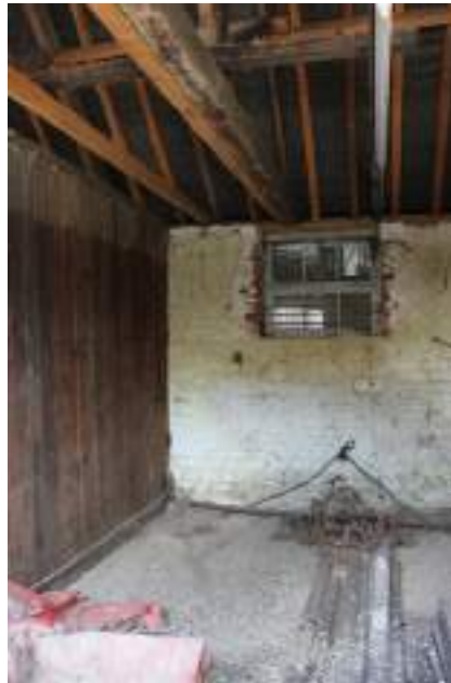
Interior of loose box with concrete floor and timber partitions
