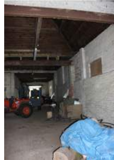
Central range looking east
