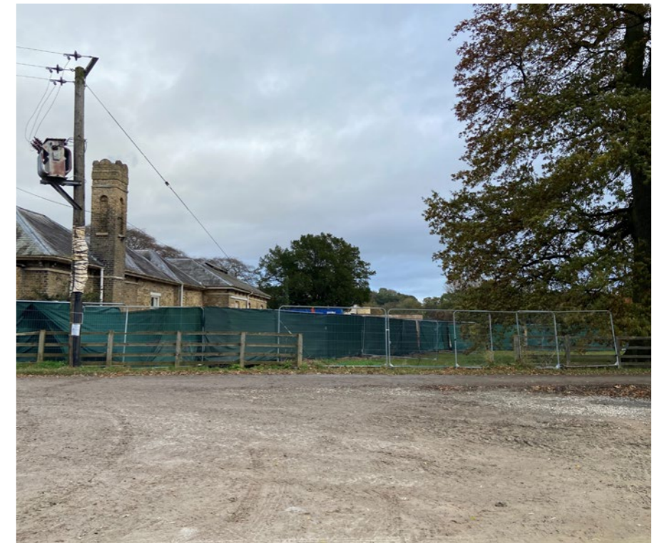
view from temporary car park
