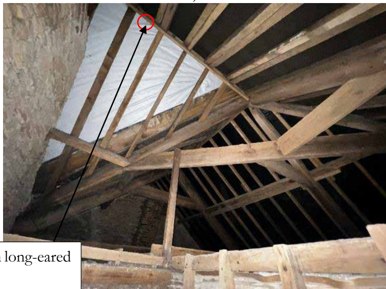
Plate 12 – stable 2, internal roof void.
