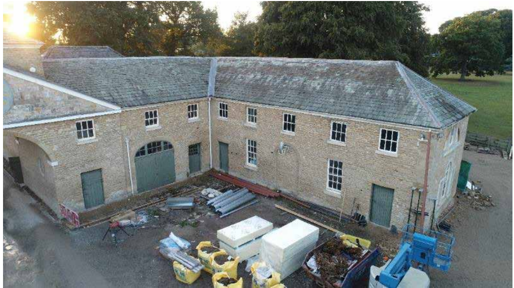
Plate 7 – Stable 2, south and east elevations.
