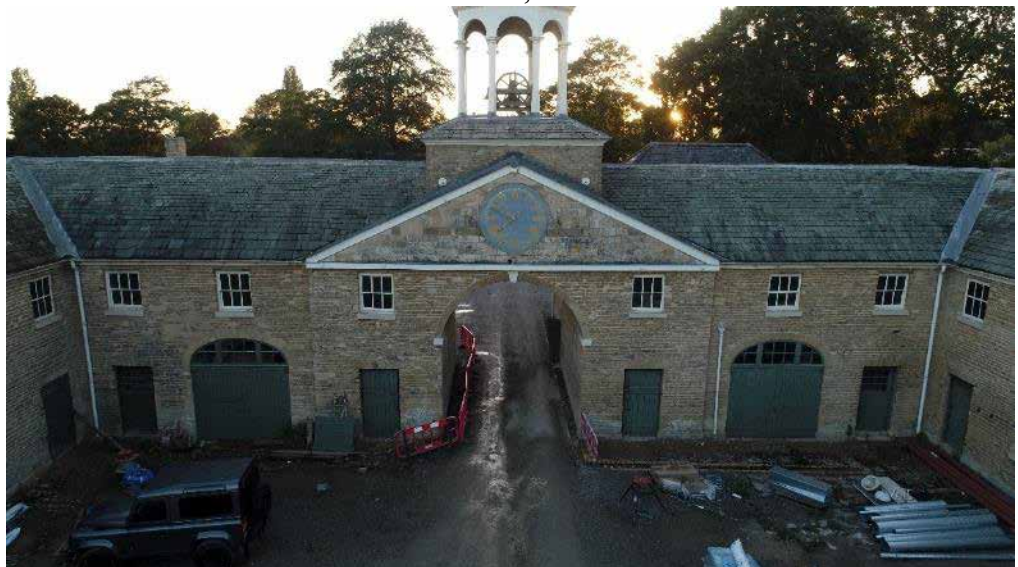
Plate 6 – Stable 2, east elevation.
