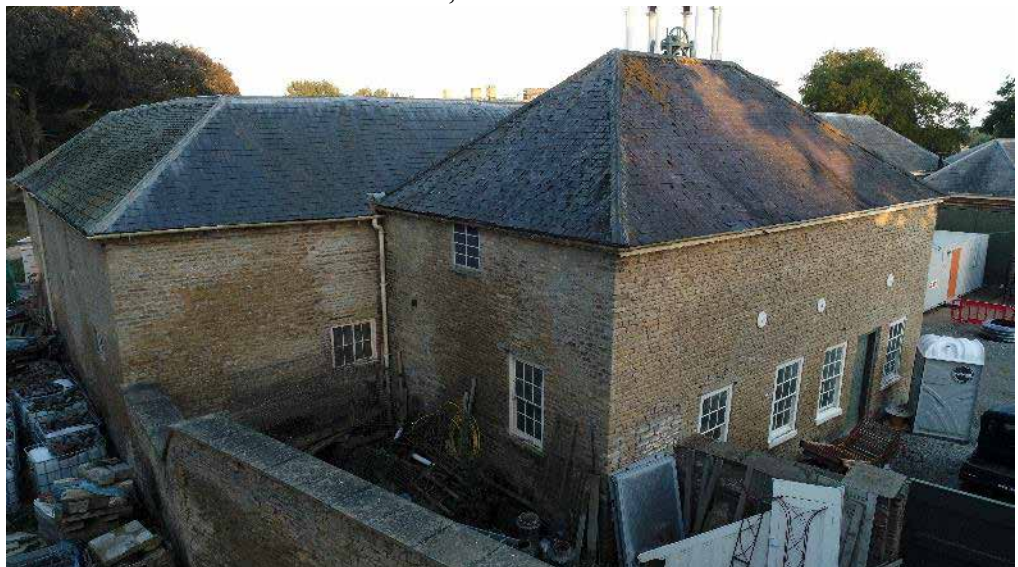
Plate 9 – Stable 2, north and west elevations.
