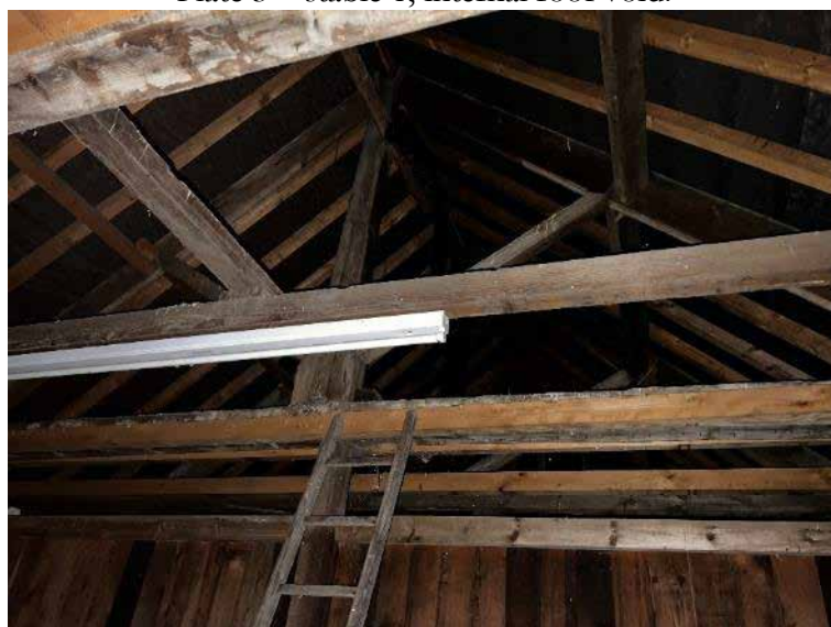
Plate 3 – stable 1, internal roof void.
