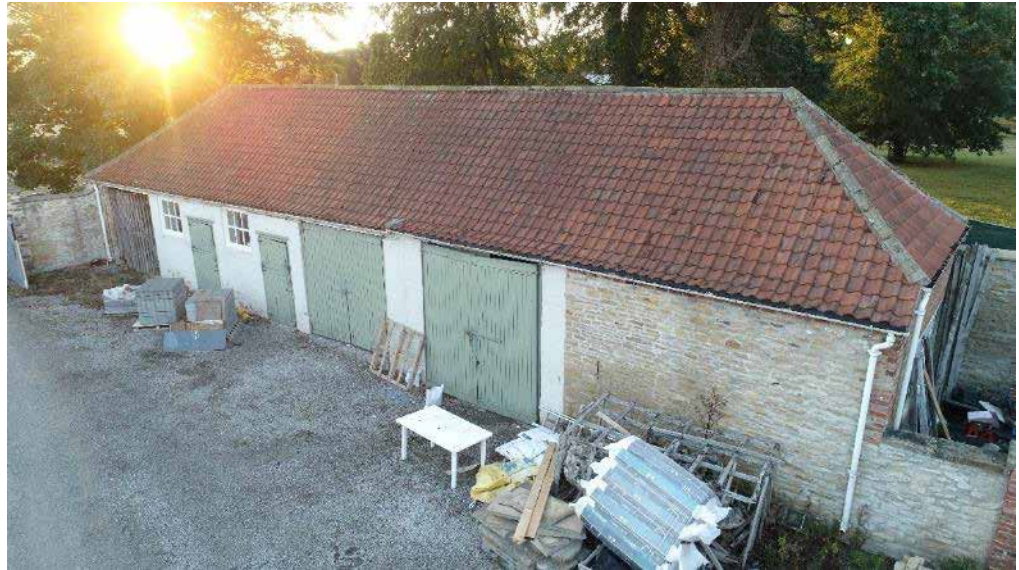
Plate 1 – Stable 1, south elevation.
