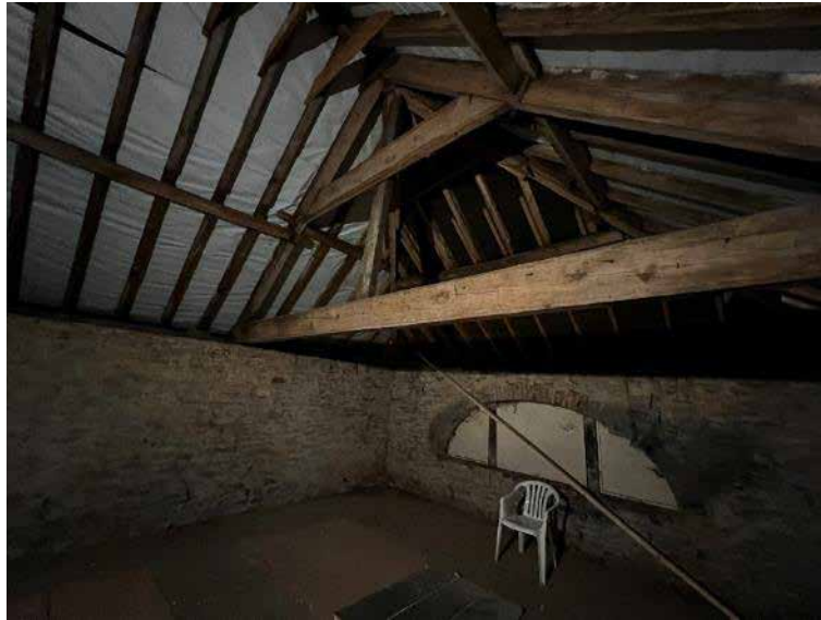
Plate 13 – stable 2, internal roof void.
