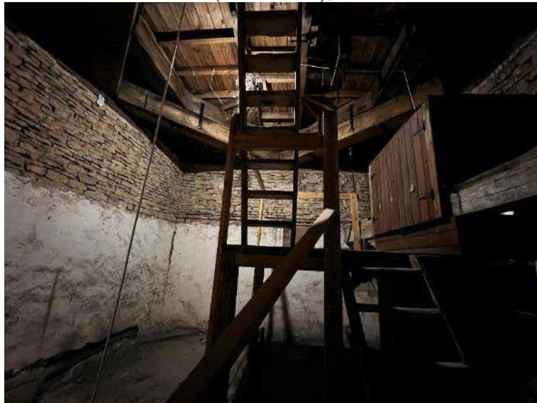
Plate 11 – stable 2 (clock tower), internal roof void.
