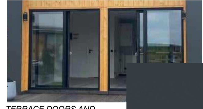
TERRACE DOORS AND WINDOWS WITH DARK GREY (RAL 7016) UPVC FRAMES
