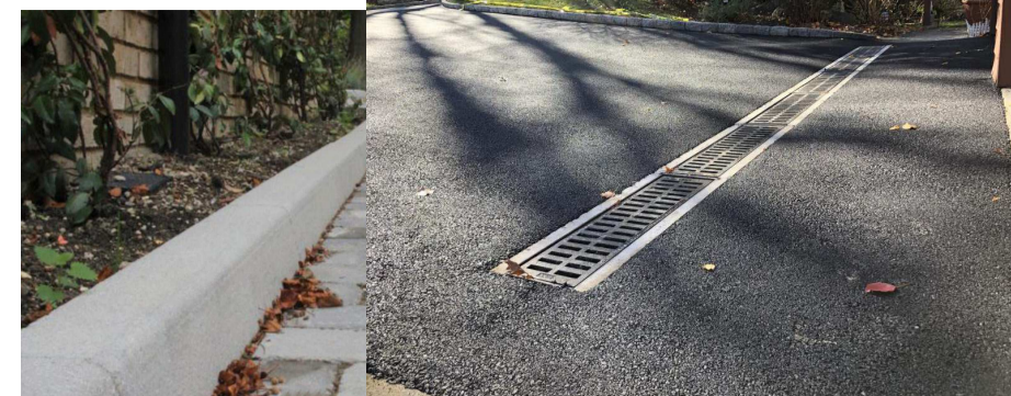
CONCRETE KERBING - 125MM HALF-BATTERED KERBS
