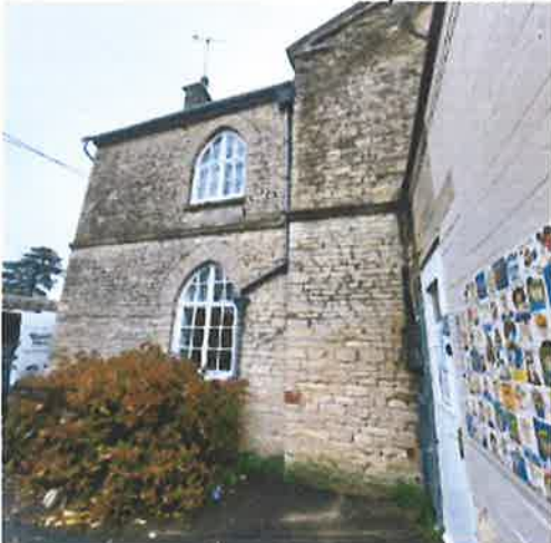
a School side wall to be pointed
