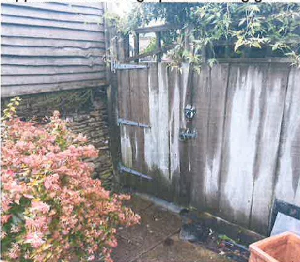
Appendix 5e Photograph of existing gate
