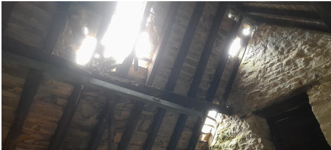
Internal view of South Roof Slope of Barn A
