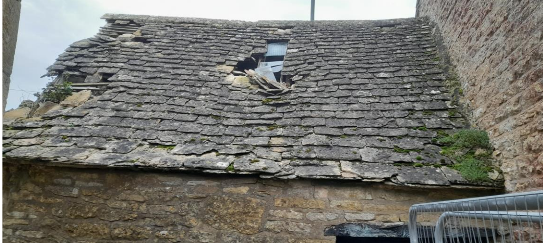
South Roof Slope of Barn A
