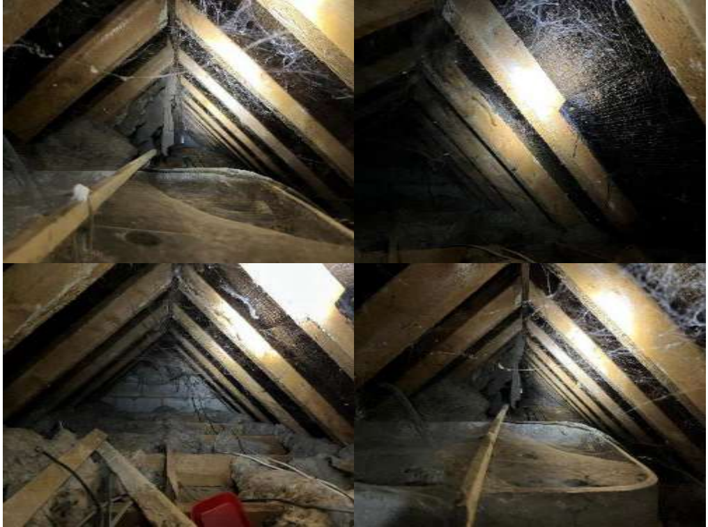
Internal main house roof void from internal PRA
