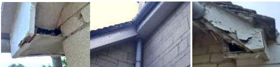
PRF 4 & 5 – gable end gap in bricks, east and west aspects respectively
