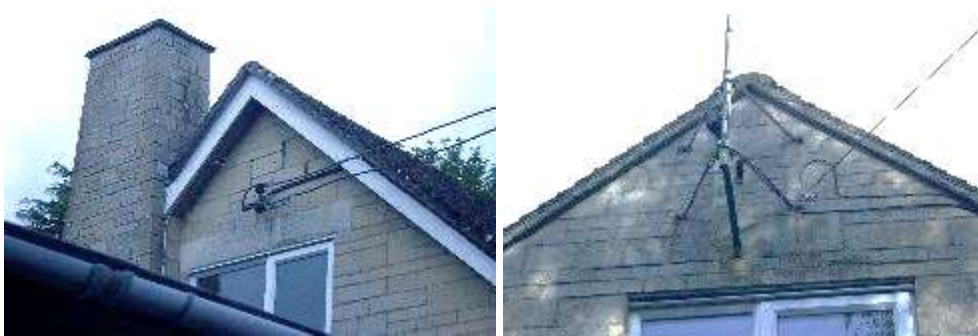
PRF 4 & 5 – gable end gap in bricks, east and west aspects respectively
