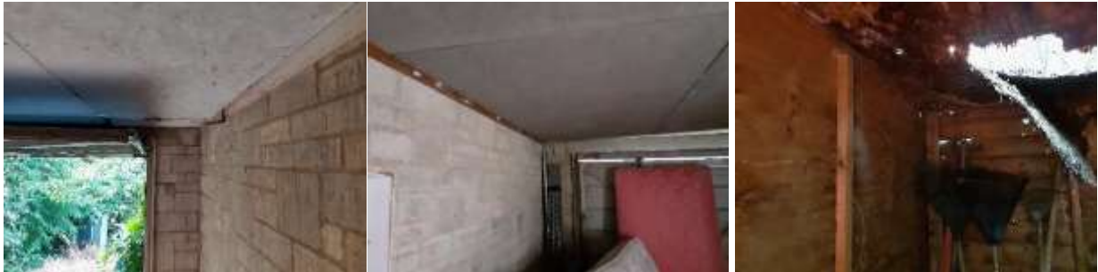
Internal double garage PRA (left, centre) and garden shed (right)
