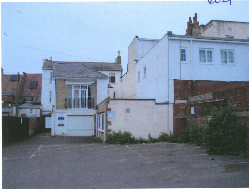
CAR PARK R/O 81/83 HIGH STREET POOLE
