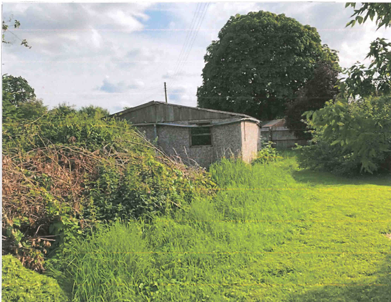
10. Additional view looking south within extensive rear garden showing disused garage building (to be removed) and large tree immediately beyond property boundary; Note: All adjacent houses are one and two storeys in height and separated away from the Cambridge Stores property
