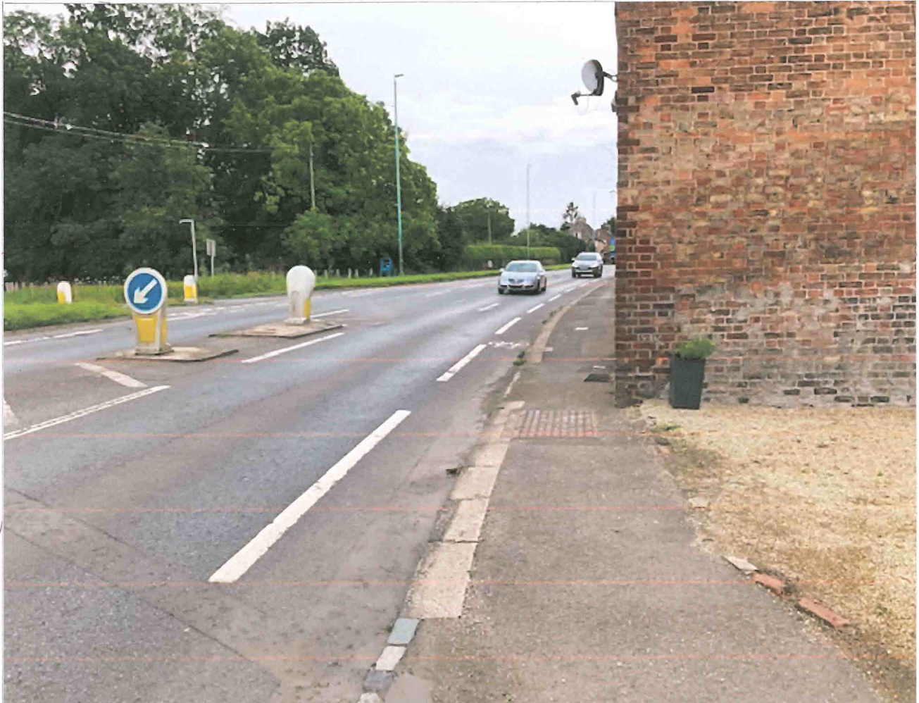
2. View looking south along A38 Bristol Road with very narrow footpath at corner beyond Bell House approx. 25m from Cambridge Stores; Note: This property restricts visibility of drivers from cars parked in front of terrace of houses particularly when reversing
