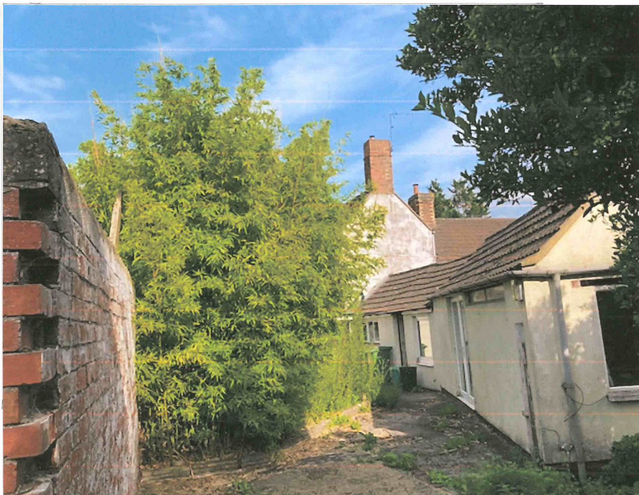
7. Additional rear view of house showing full extent of elongated rear ground floor addition as well as masonry wall to adjoining neighbour's garden (to left); Note: As described in photograph 6. proposal to completely remove rear addition, form walled garden to house with separate access under part of house to large rear garden (not in view) to two new two storied dwellings (See drawings 1 and 2)
