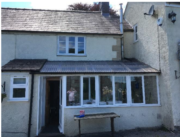
Existing lean-to utility area
