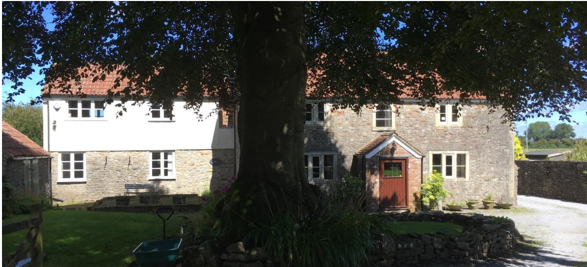
Front elevation – photo taken from public highway.
