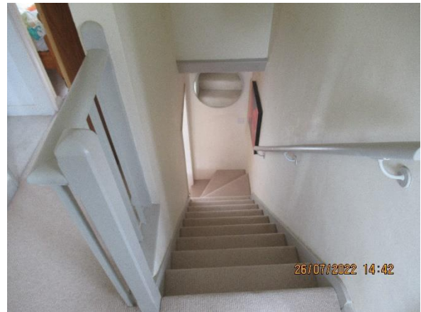
Annex – Existing modern staircase
