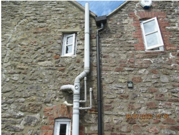
LHS – front portion of cottage. RHS later addition difference in stone mix used for walling.
