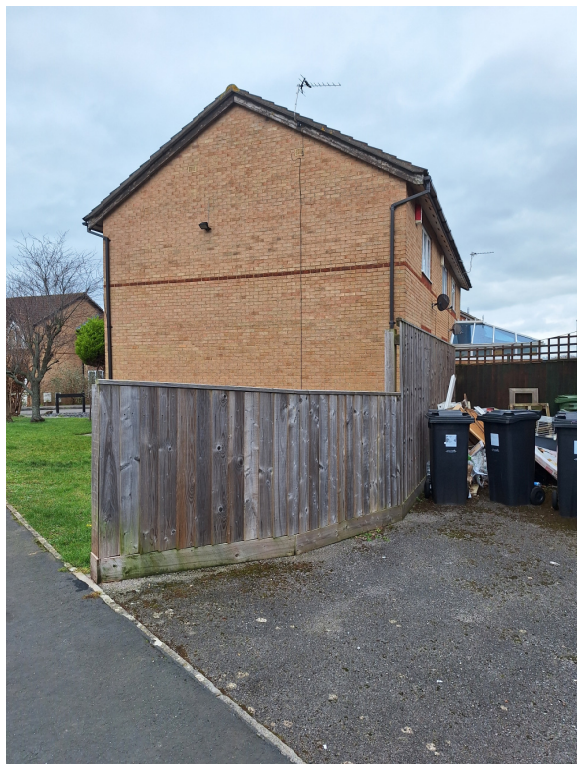
Existing fence to southern boundary
