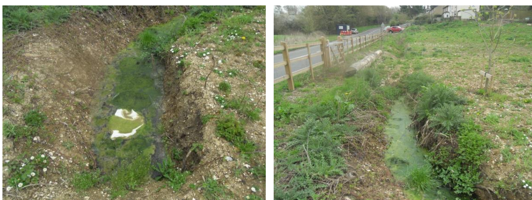
Ditch holding water 15 th April 2018 and still inundated on 9 th June 2018
