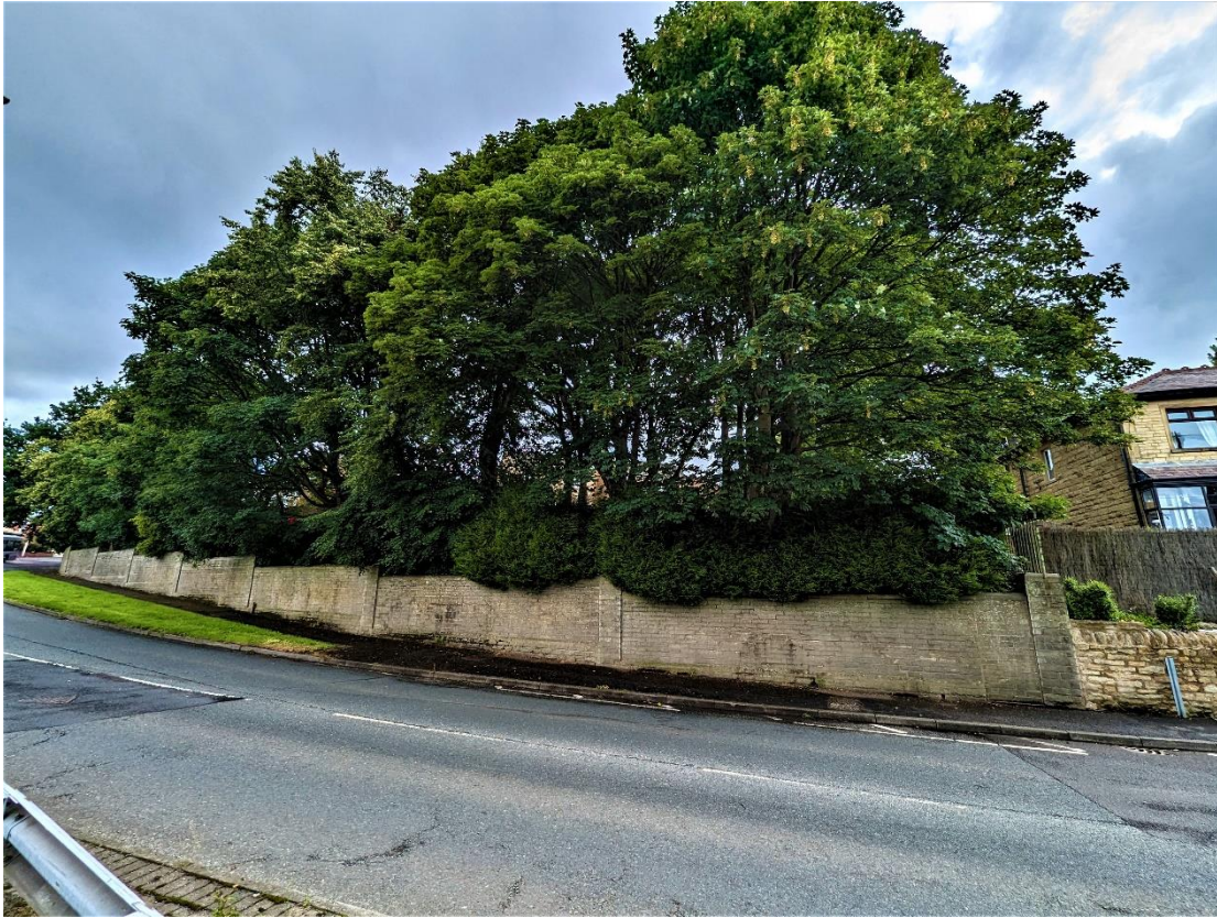
Photograph 01 – General view of the front face of the retaining wall.
