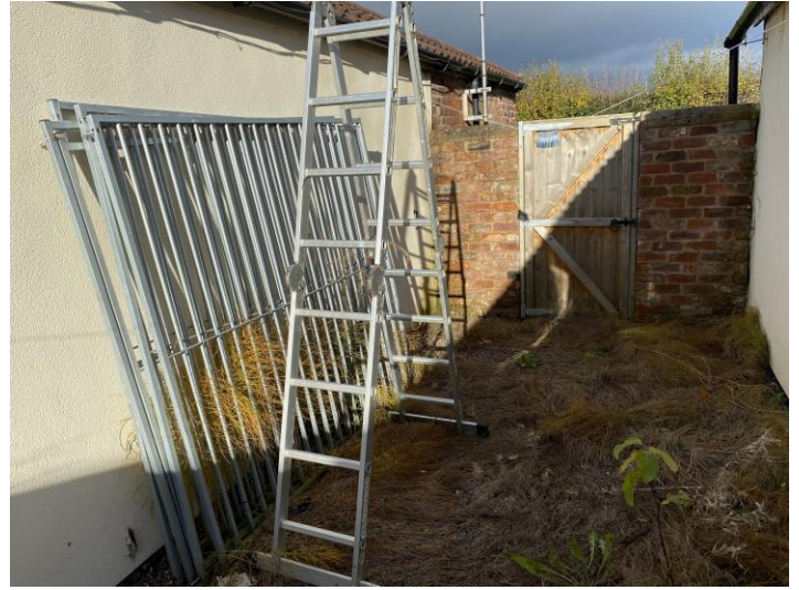
Image showing No.6 Edge Grange Barns from the rear courtyard
