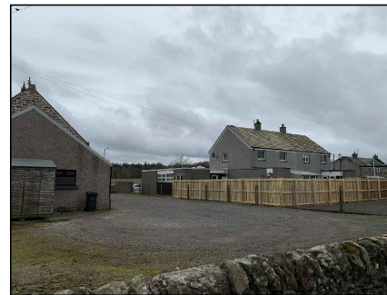
East & North Elevation - street view
