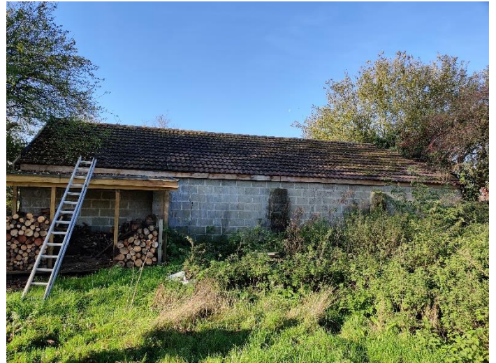
Photo 2 East elevation of barn
