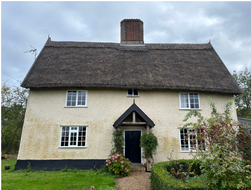
West Elevation of Perkins Farm
