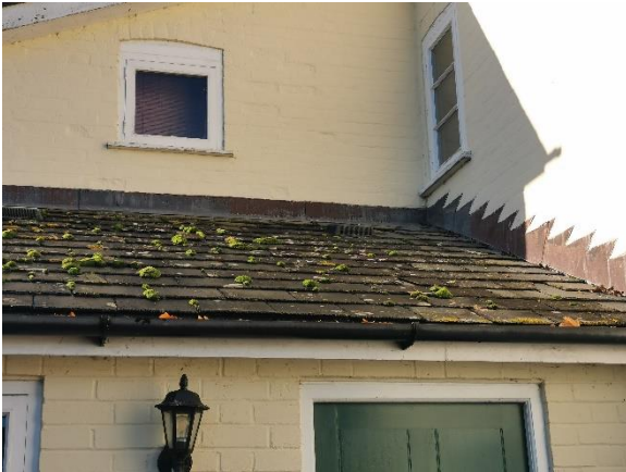
Roof tiles on eastern roof section.
