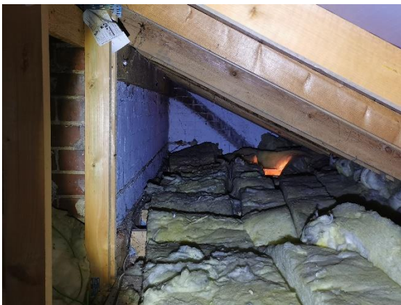
Internal loft space.
