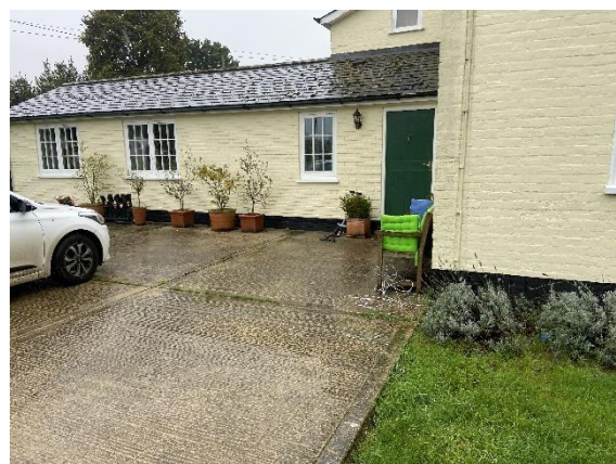
Concrete hardstanding to the northeast of the house
