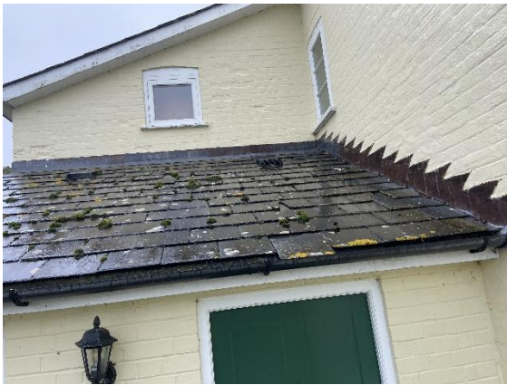
Broken tiles and minor lifted tiles on the eastern single-storey wing of the house. (Looking southwest)
