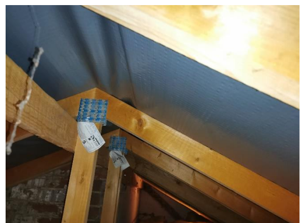
Internal roof lining.
