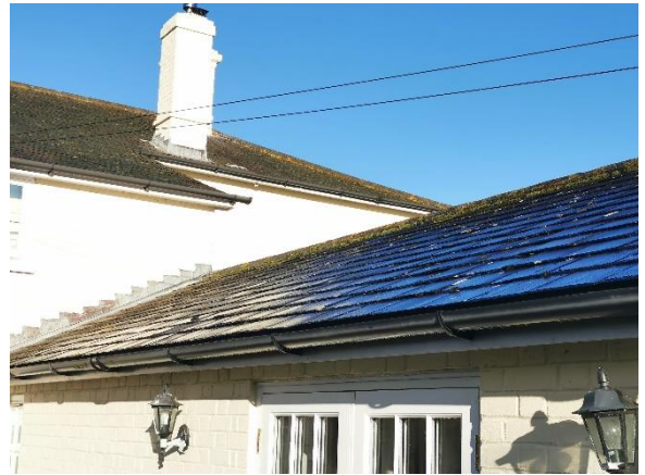
Roof tiles on western roof section.
