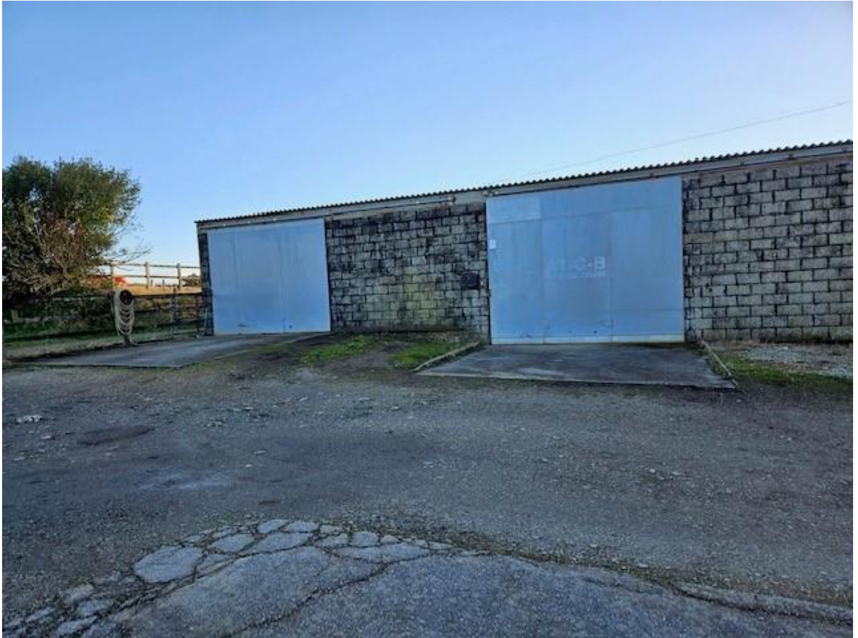
Northern end of western elevation
