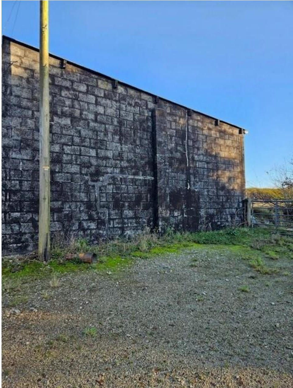
Northern end of eastern elevation
