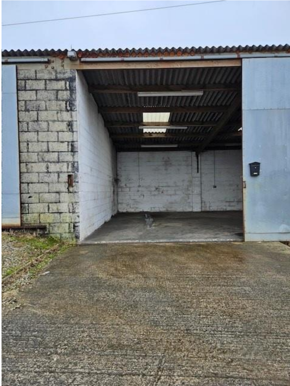
Entry doors in western elevation
