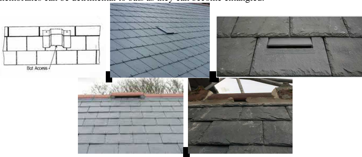
Figure 6: Examples of bat access slates (top) and modified ridge tiles (bottom).
