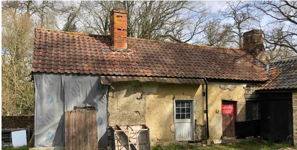
South elevation showing remains of greenhouse flashing, (greenhouse now demolished)
