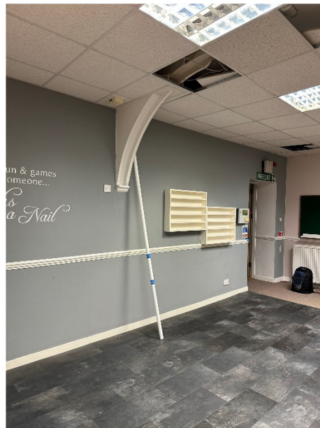
06_Interior arched steelwork
