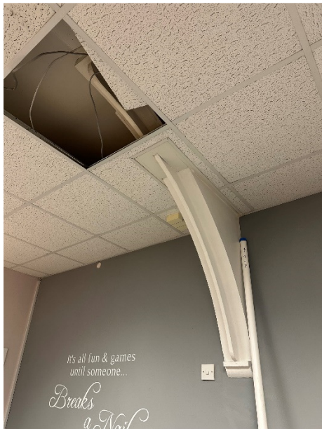
05_Interior arched steelwork
