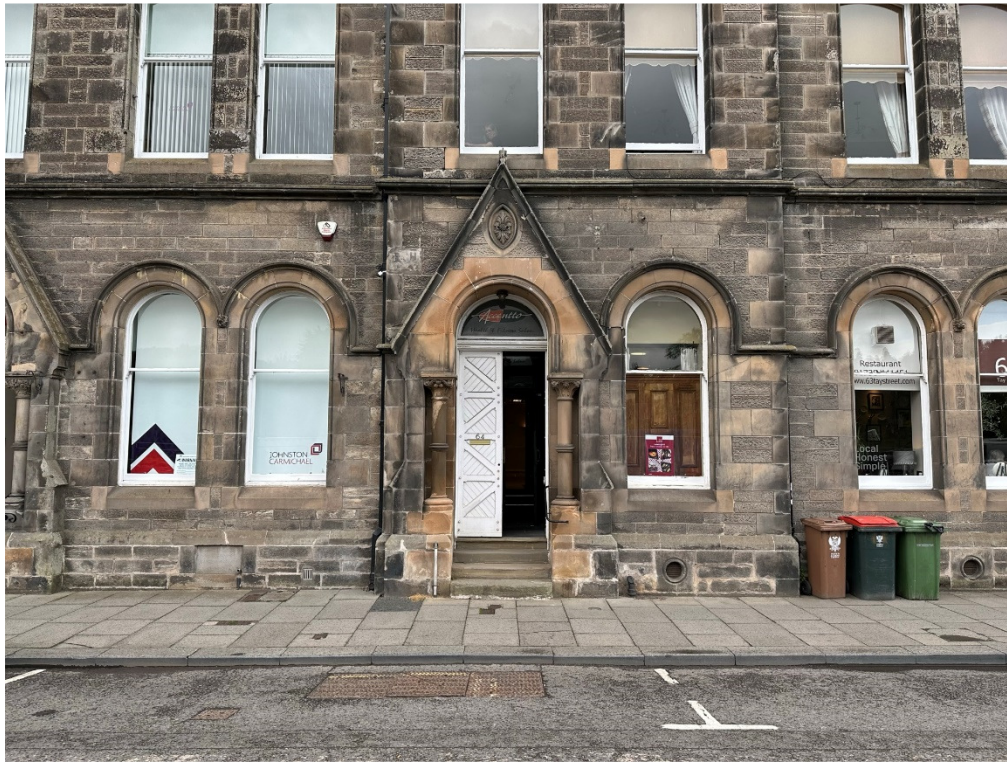
01_East façade at Tay Street
