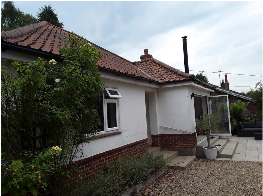
Figure 5 – Looking southwards at the existing dwelling.
