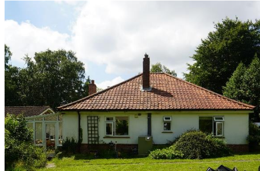
Figure 3: Existing Rear Elevation
