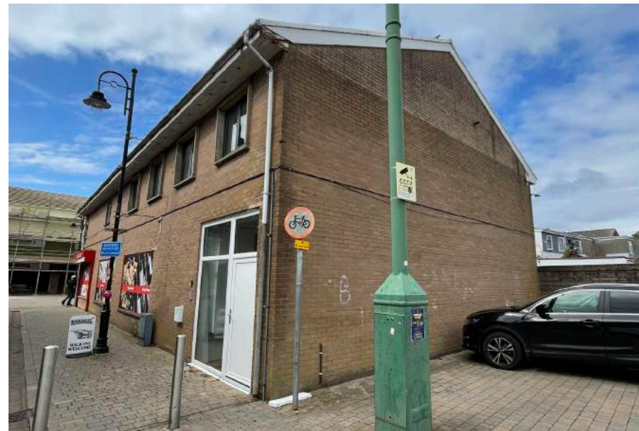
Rear view of Holman House
