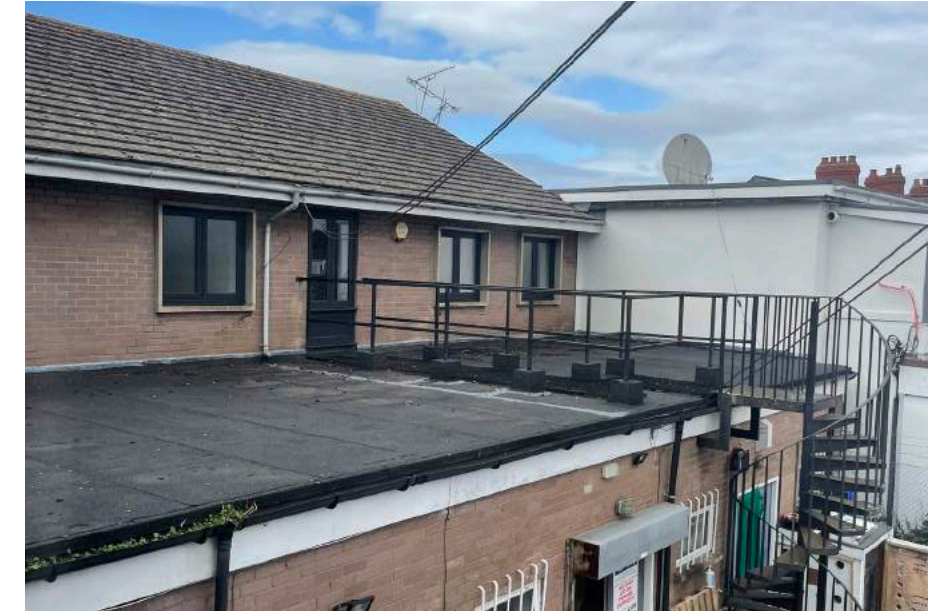
Flat roof at rear of Holman House
