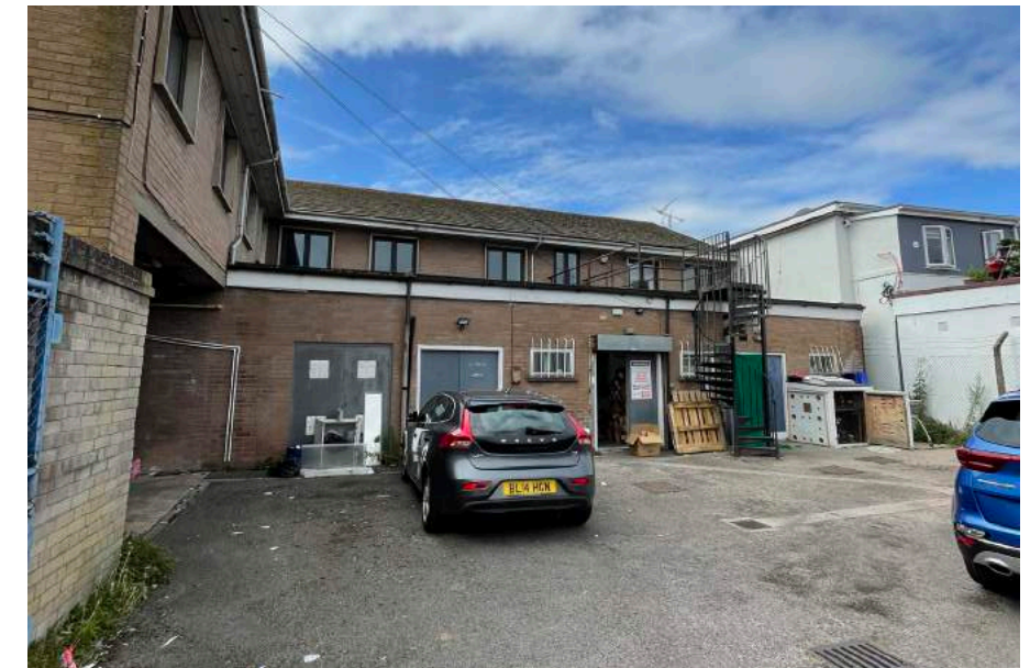
Rear parking and services for commercial units at ground floor
