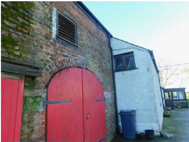
PHOTO 7 View Along Northern Barn Elevation
