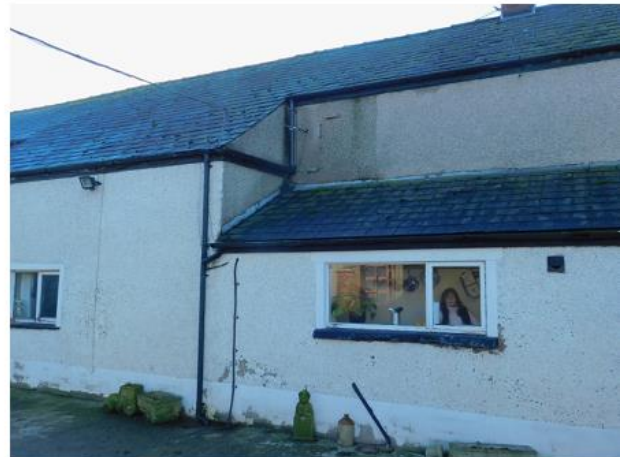
PHOTO 12 North-Western View of Main House
