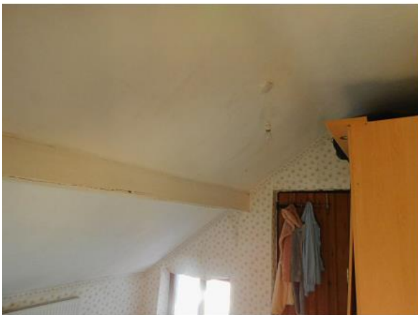
PHOTO 29 Underside of Central Main Building Roof
