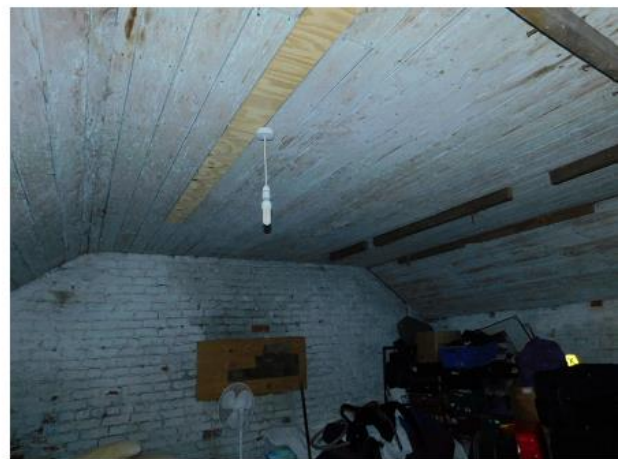
PHOTO 30 Underside of Southern Main Building Roof
