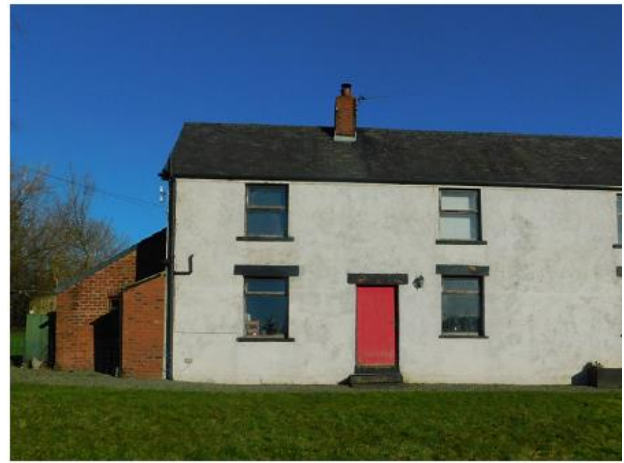
PHOTO 22 South-western Corner of Main Building
