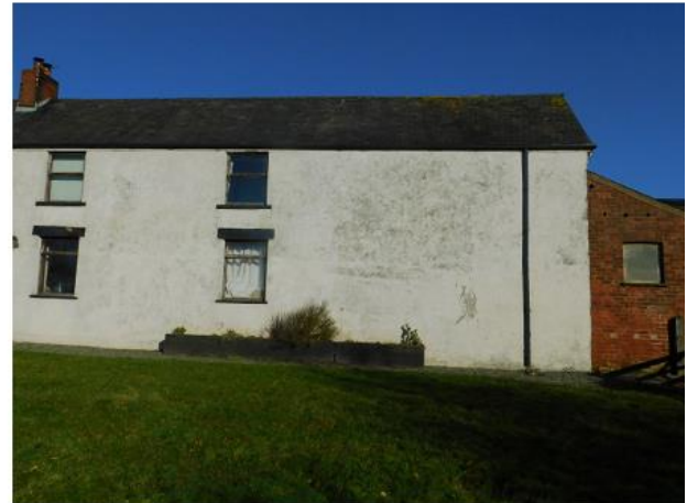
PHOTO 24 South-eastern Corner of Main Building
