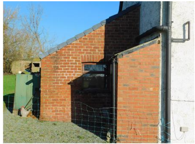
PHOTO 20 Southern Elevation of Outbuildings
