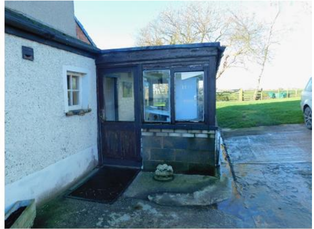
PHOTO 14 Eastern Elevation of Conservatory
