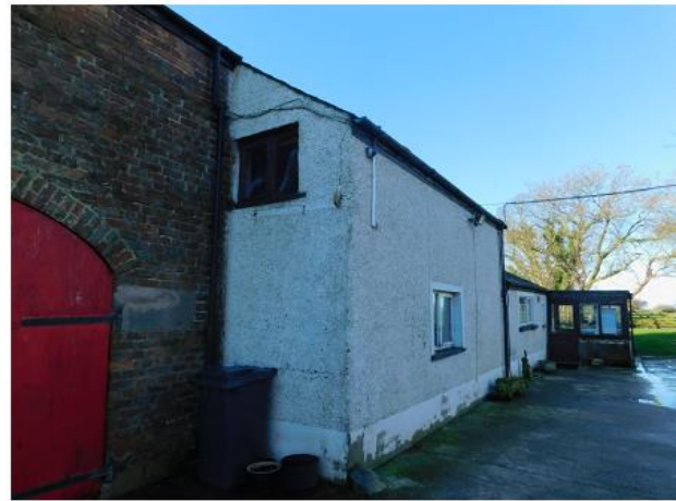
PHOTO 10 North-eastern Corner of Main Building
