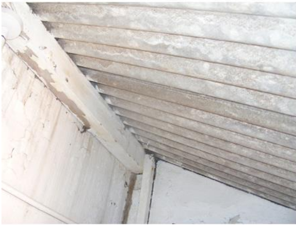
PHOTO 21 Underside of Sloping Roof of Outbuilding
