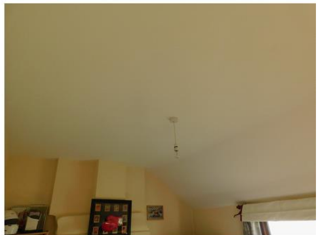
PHOTO 28 Underside of Northern Main Building Roof
