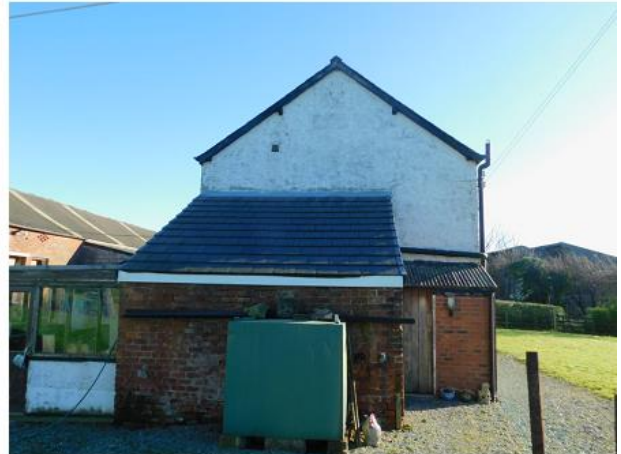
PHOTO 18 Eastern Elevation of House and Outbuildings
