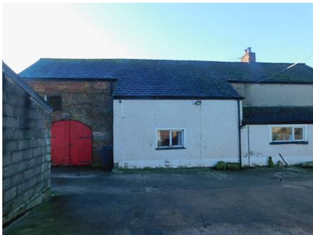
PHOTO 11 Northern Elevation of Main Building
