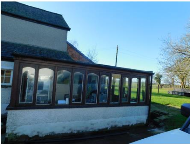
PHOTO 15 Northern Elevation of Conservatory
