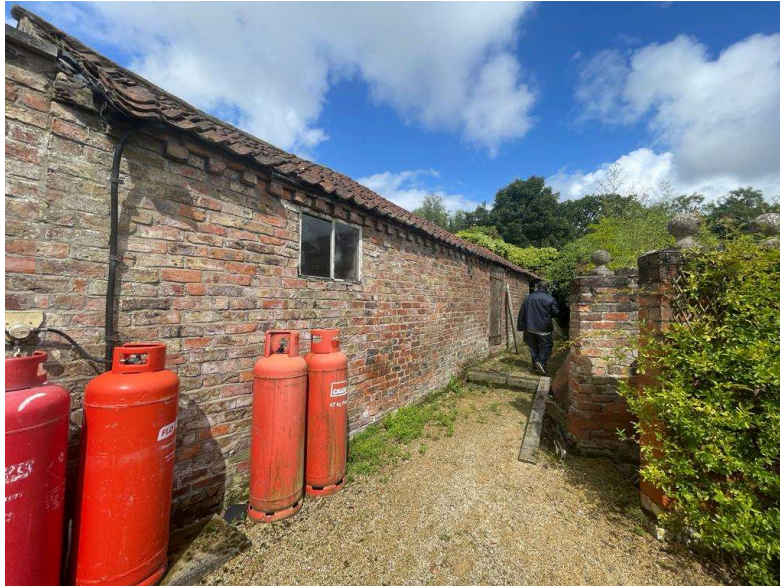
The current state of Building A
