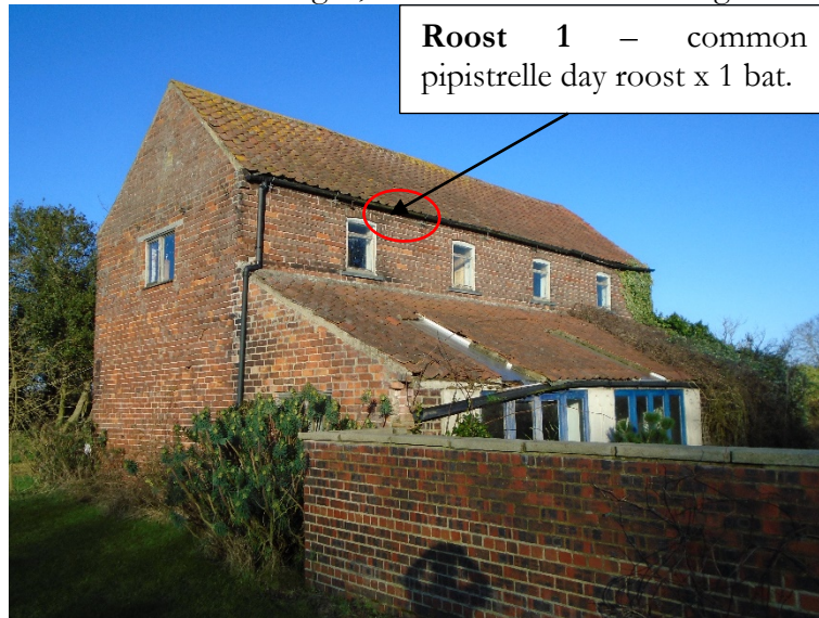
Plate 4 – outbuilding B, south elevation and west gable.
