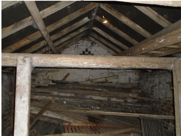
Plate 3 – outbuilding A, internal roof structure.
