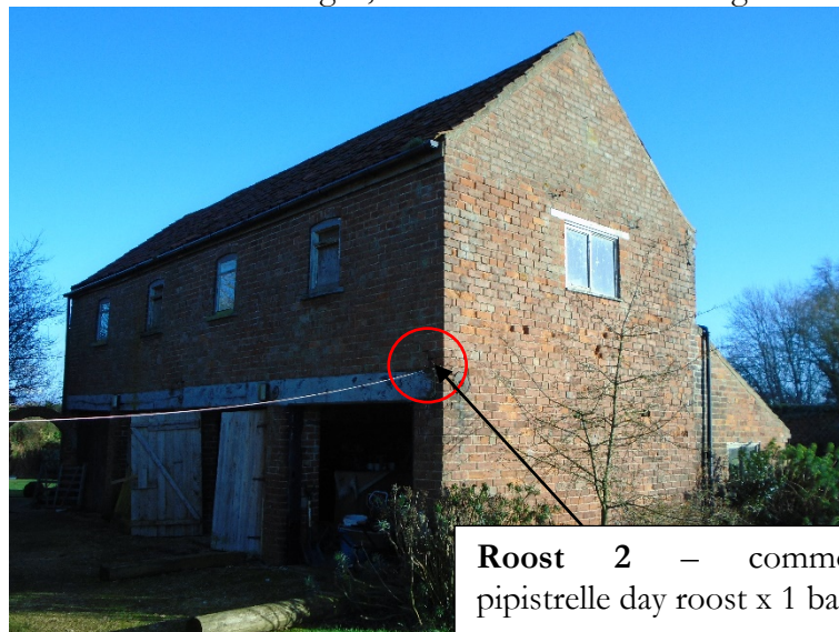
Plate 5 – outbuilding B, north elevation and west gable.
