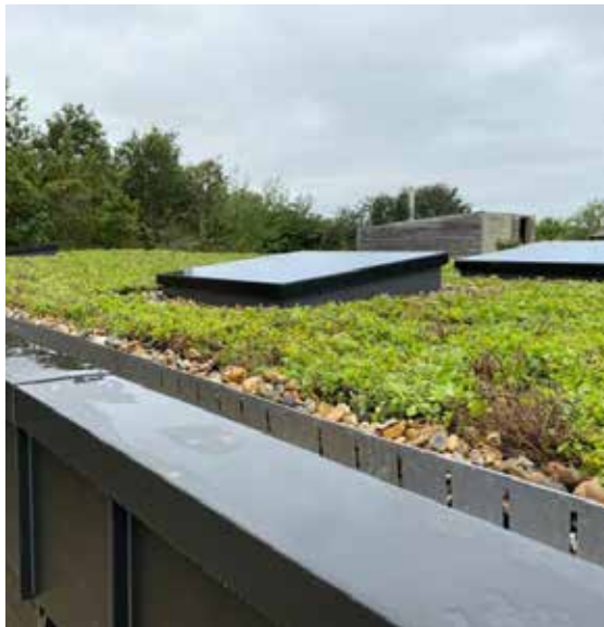
Wildflower sedum roof with dark aluminium trims and flat glass roof lights
