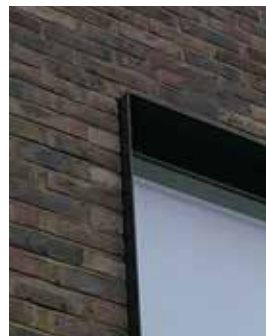
Modern format brickwork with thin PPC metal coping, PPC metal lining to window / door openings, zinc cladding panels adjacent to rear sliding doors & main entrance
