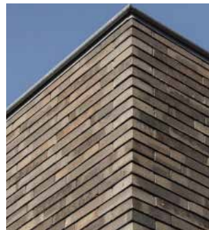
Modern format brickwork with thin PPC metal coping, PPC metal lining to window / door openings, zinc cladding panels adjacent to rear sliding doors & main entrance
