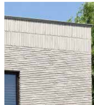
Modern format brickwork with thin PPC metal coping, PPC metal lining to window / door openings, zinc cladding panels adjacent to rear sliding doors & main entrance
