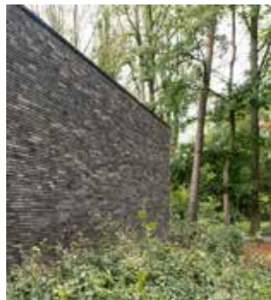
Modern format brickwork with thin PPC metal coping, PPC metal lining to window / door openings, zinc cladding panels adjacent to rear sliding doors & main entrance
