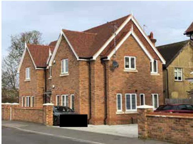
Rear corner view of No.257 with access to parking area
