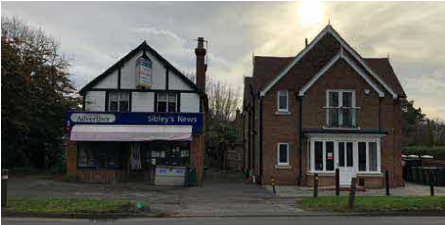
Primary front view of site and No.257
