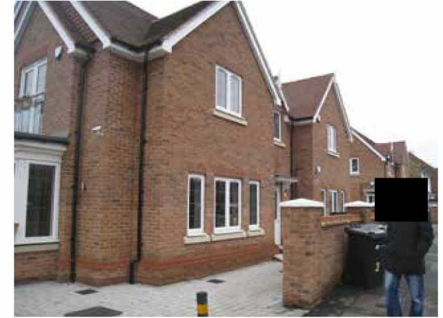
Hard landscaped area for bin stores and brick boundary walls
