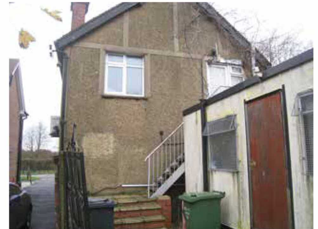
Rear elevation and metal staircase to existing building
