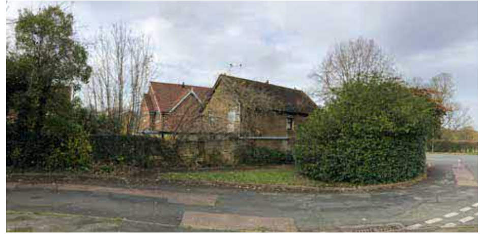
Side elevations onto pavement to the East (No257 in background)
