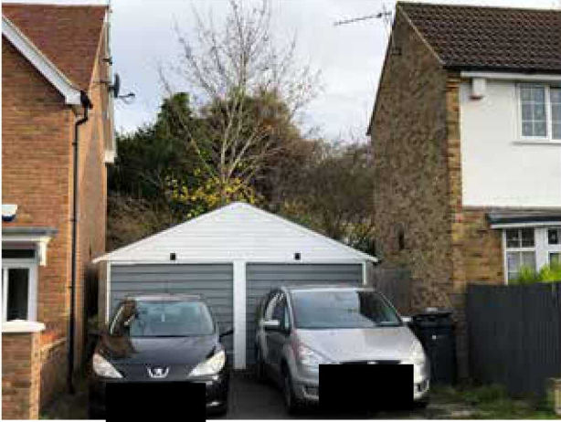
Garages and parking to Englands House
