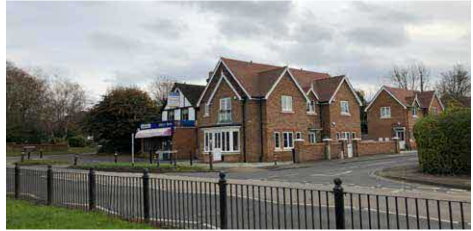
View of site and No.257 from Guildford Road
