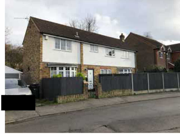
Front view of Englands House facing onto Norwood Road
