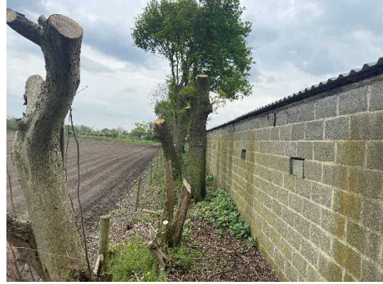
Photograph 4 - Line of broadleaved trees along the western boundary.
