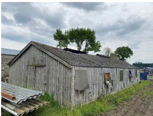
Photograph 10 – Showing the northern and eastern elevations of B2.
