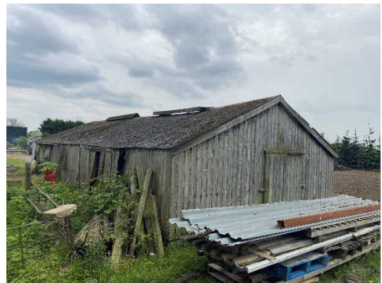
Photograph 9 – Showing the western and southern elevations of B2.
