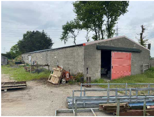
Photograph 6 – Showing the western and southern elevations of B1.
