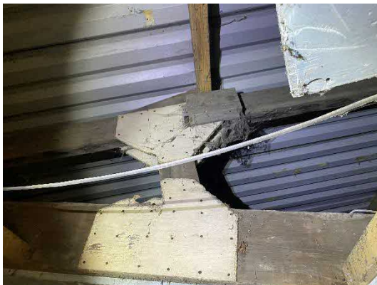
Photograph 8 – An example of the timber sheeting at timber roof joists.
