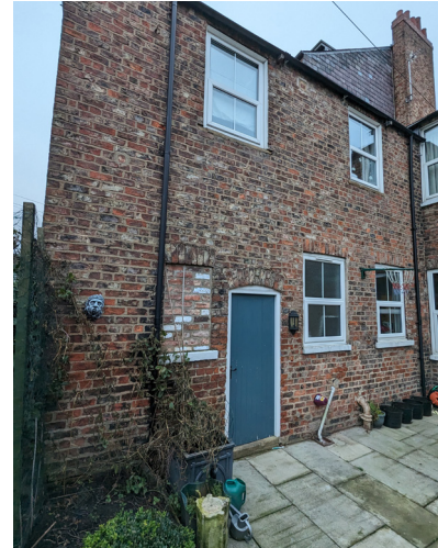
Side of rear extension
