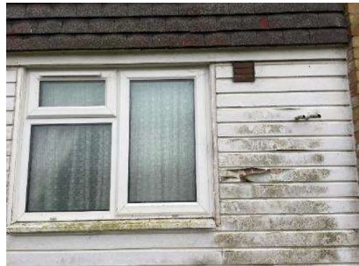
Fig 13 – Vent through timber cladding.
