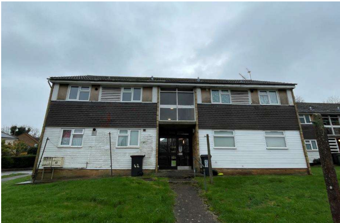
Fig 03 – Rear view of Block 42-44 from car park (North Elevation).
