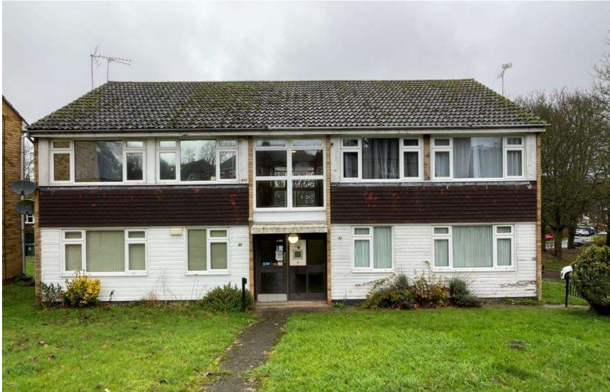
Fig 02 – Front view of Block 42-44 from Pickford Road (South Elevation).
