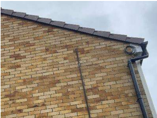
Fig 25 – Detail view of verge tiles.
