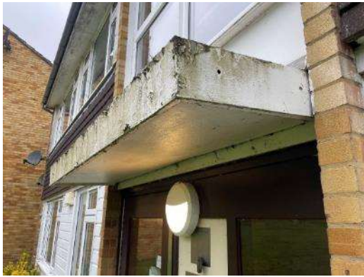
Fig 10 – Entrance canopy condition.
