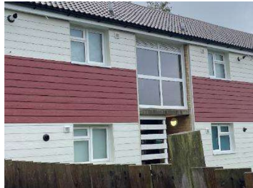
Fig 26 – Vents through Cedral cladding.
