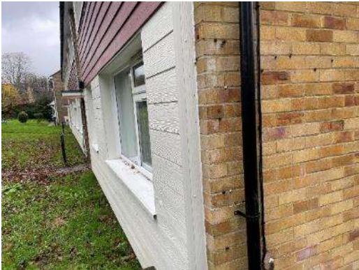
Fig 21 – View of Cedral cladding extending out.
