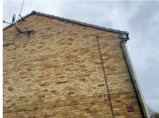
Fig 24 – Side elevation with verge tiles.
