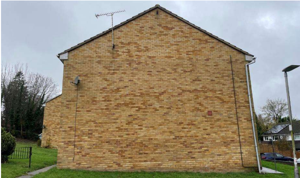
Fig 04 – Side view of Block 42-44 (East Elevation).
