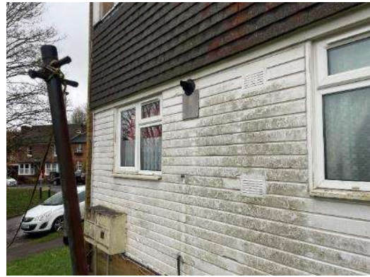
Fig 11 – Timber cladding condition at rear.
