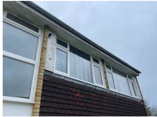
Fig 07 – Infill panels condition at front.
