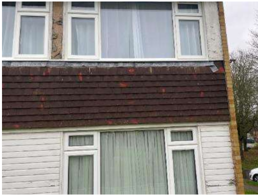
Fig 08 – Tile hanging and flashing condition.
