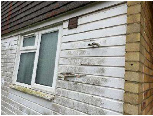
Fig 06 – Timber cladding condition at front.
