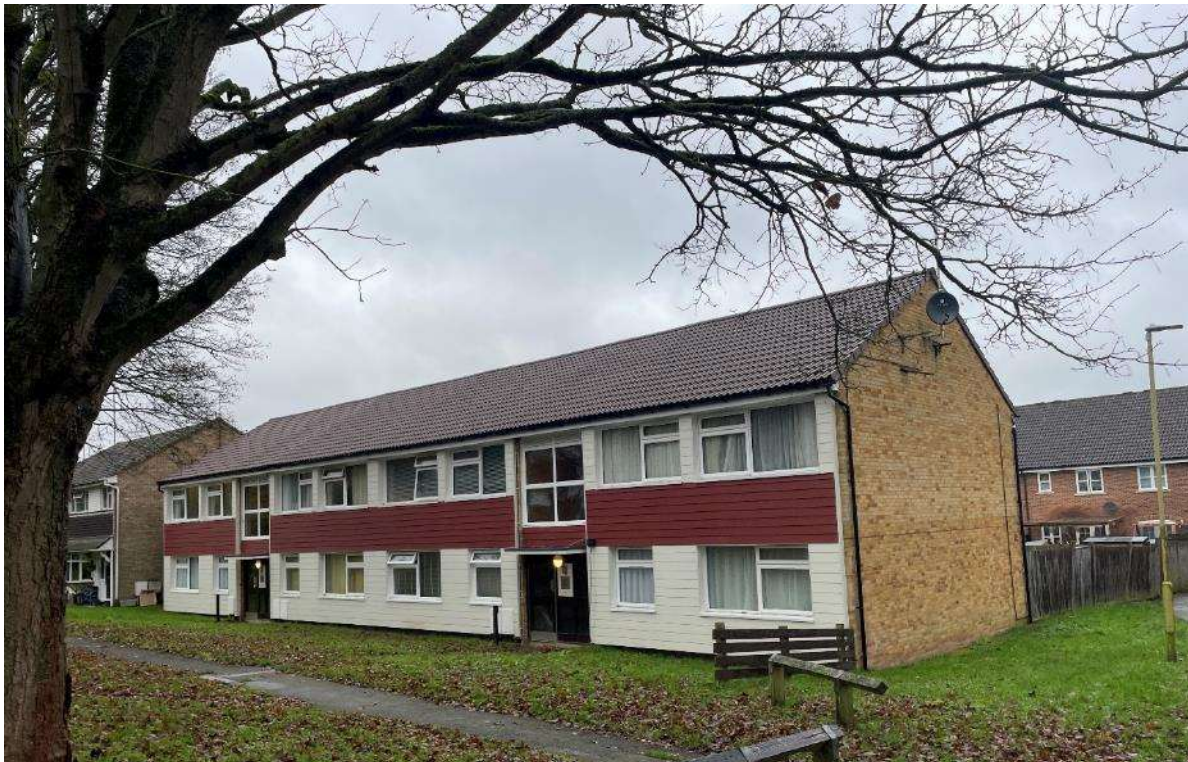
Fig 14 – View of refurbished front elevation of Block 6-9A Sebright Road.
