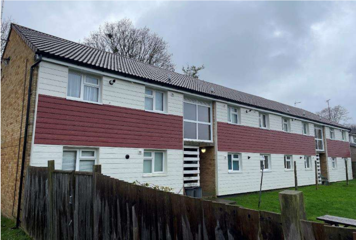
Fig 15 – View of refurbished rear elevation of Block 6-9A Sebright Road.
