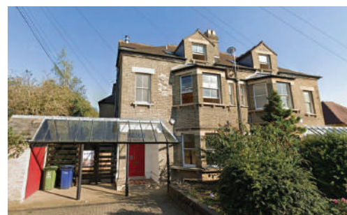
Fig 2.3: View towards houses immediately opposite showing their loft dormers to front and side.
