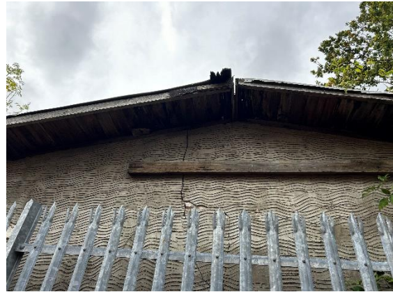
Photo 2 – Access points on Building B4
